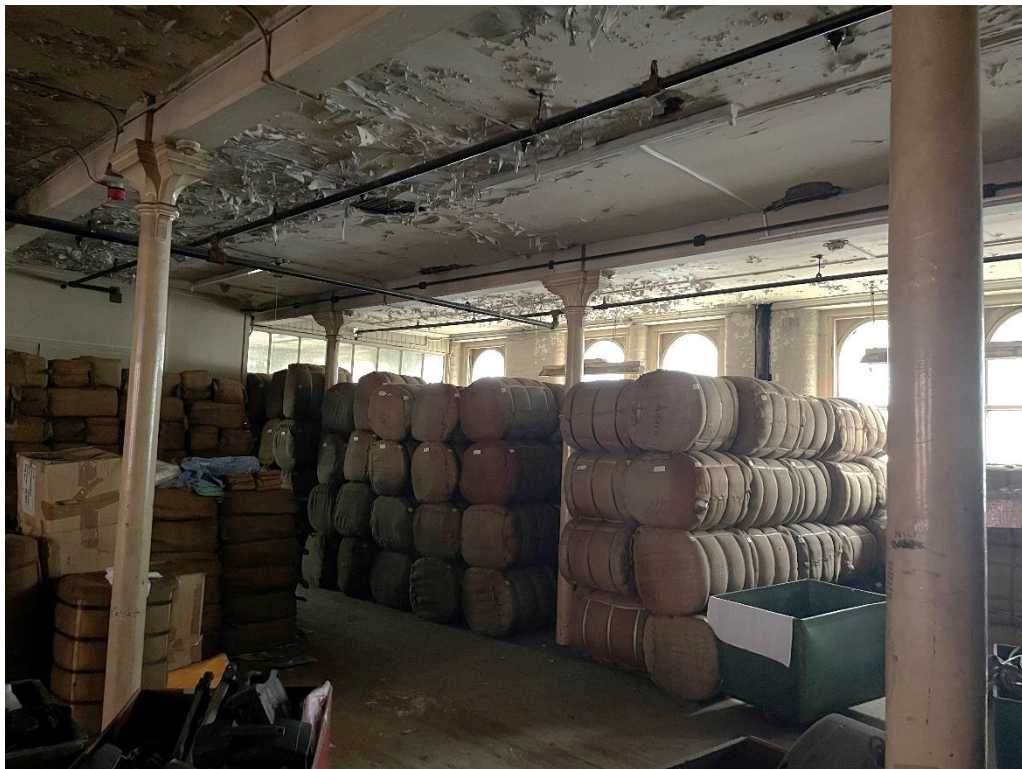
Figure 4.5: View of the interior of 42 Bloom Street at second floor level
