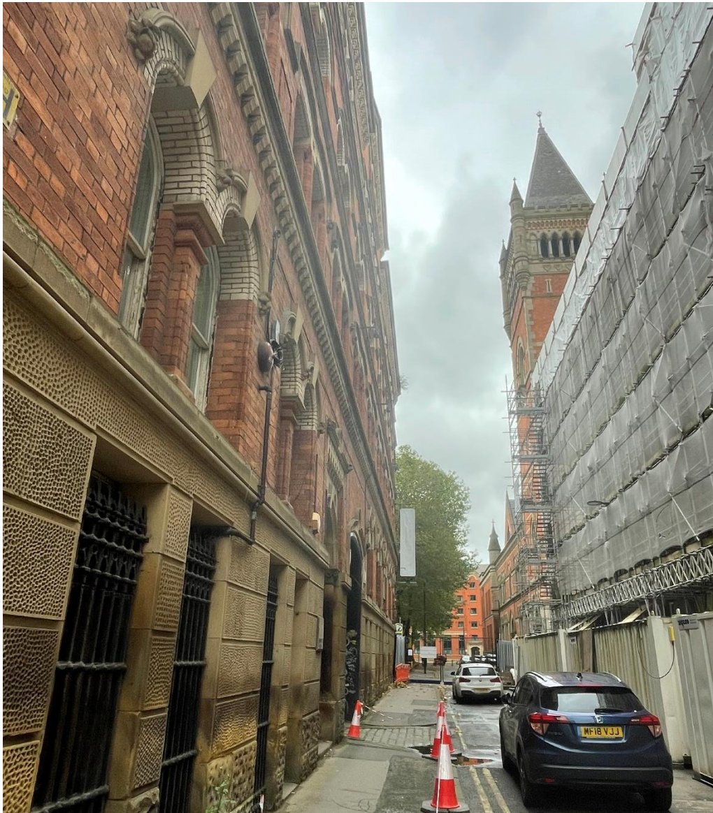
Figure 4.2: View north east on Bloom Street. The south east elevation of 42 Bloom Street is visible in the left hand side of the image
