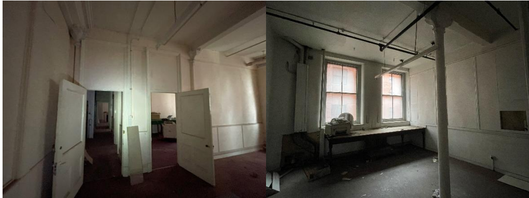
Figure 4.6: Views of the former ground floor offices in 8 Minshull Street
