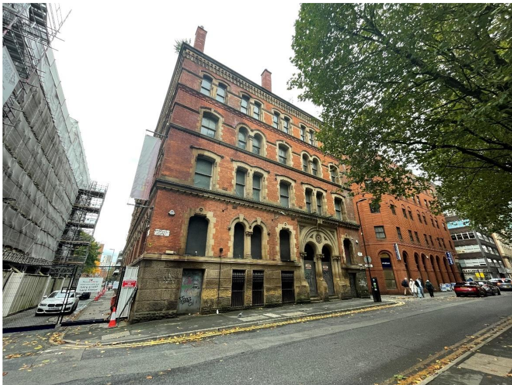
Figure 4.1: View of the principal (north east) elevation of 8 Minshull Street from the east on Minshull Street
