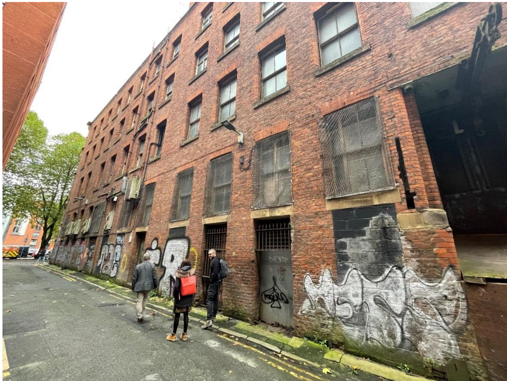
Figure 4.4: View of the north west elevation of 8 Minshull Street and 42 Bloom Street from the north west on Hart Street
