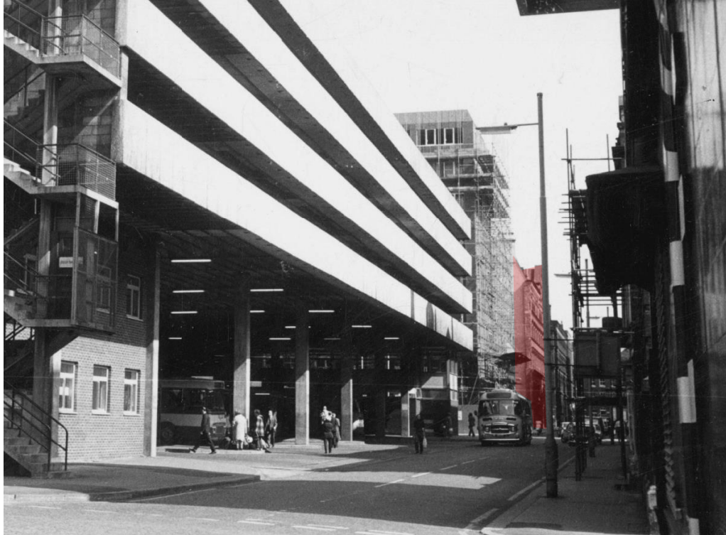
Figure 2.7: Photograph facing north east along Bloom Street towards the Site, 1973 (Manchester City Council)
