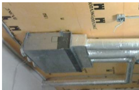
Figure 13 - Typical Ducted Fan Coil Unit
