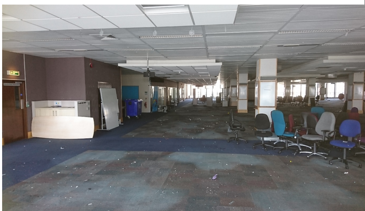
04-18 View looking west across open plan office with separate offices and meeting rooms to the left hand side.
