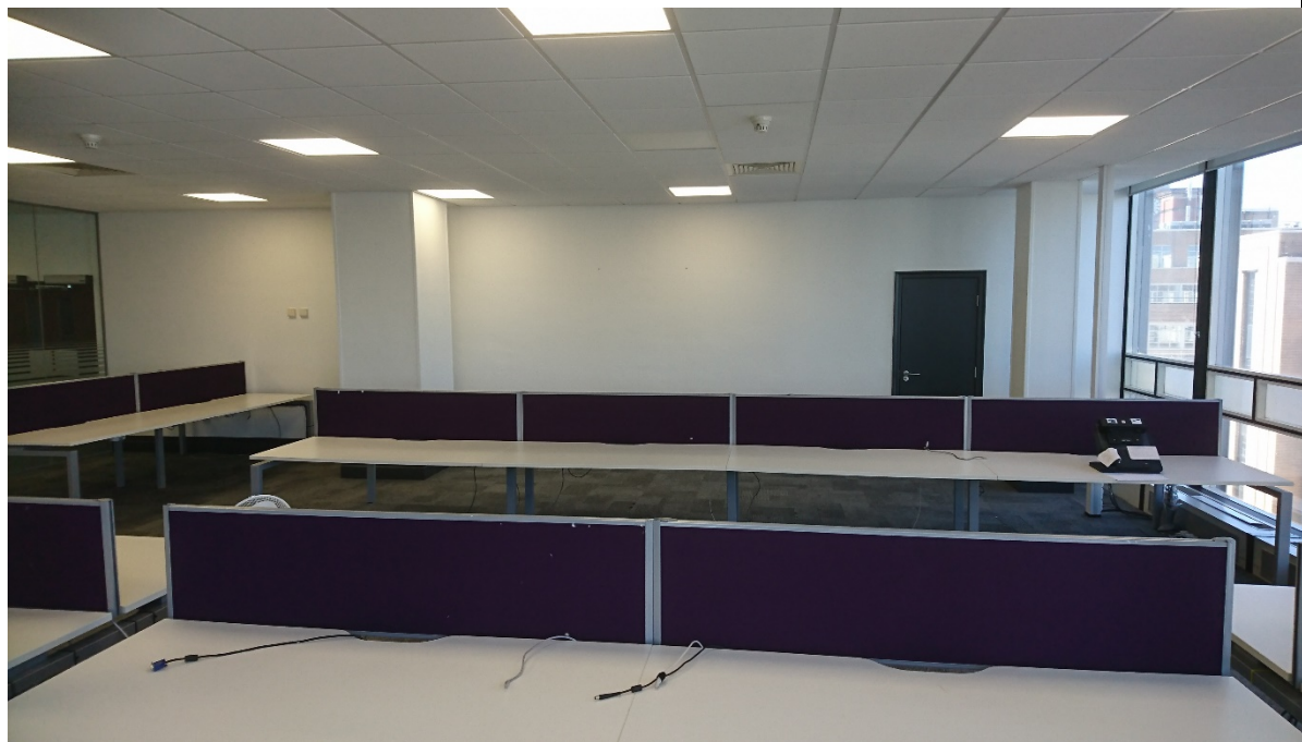
04-09 View looking south towards partitioning, desks and ceiling within office space.
