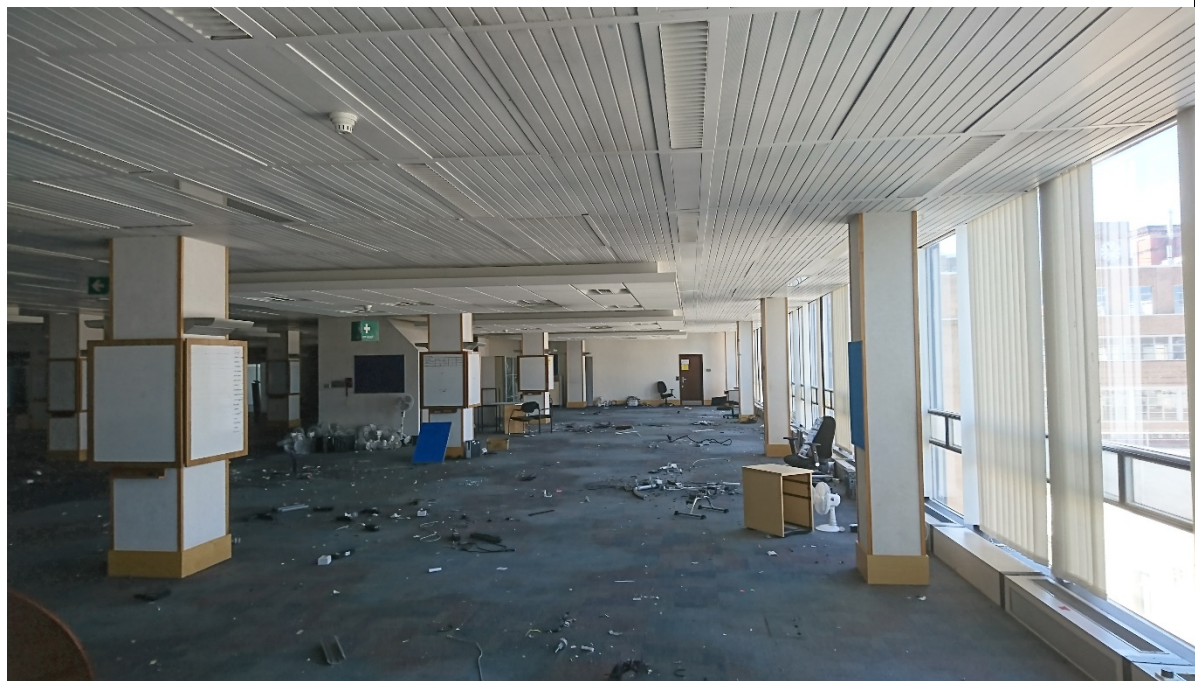
04-13 View looking south within open plan office space.
