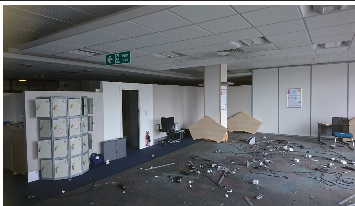
04-24 View of open plan office space with full and half height non-original partitions, also showing the inserted lower lighting unit below the original ceiling height.
