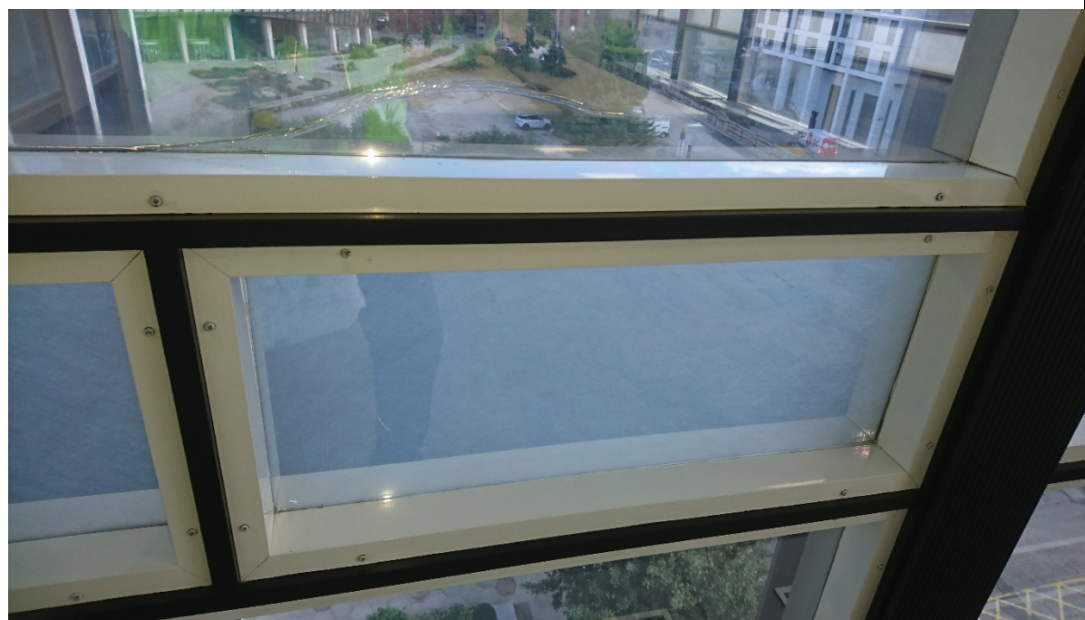
04-29 Detail of the curtain walling and glazing that has had the timber bead replaced with a painted aluminium bead around each piece of glazing.
