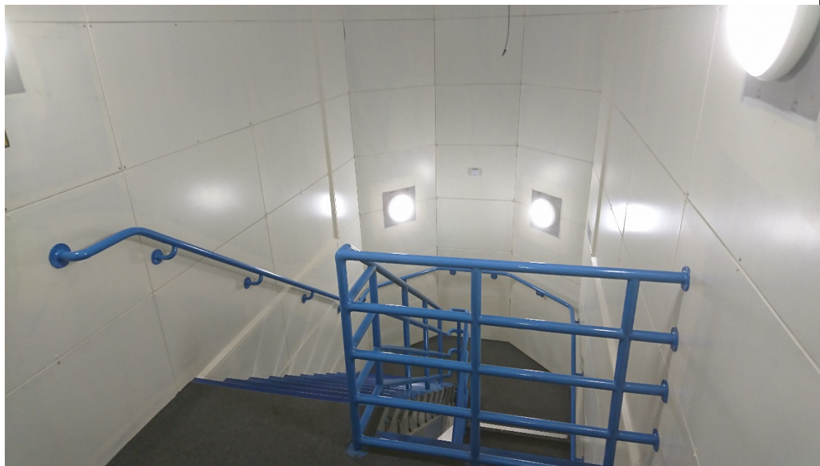
04-35 View from the top of the inserted north-east stairwell.
