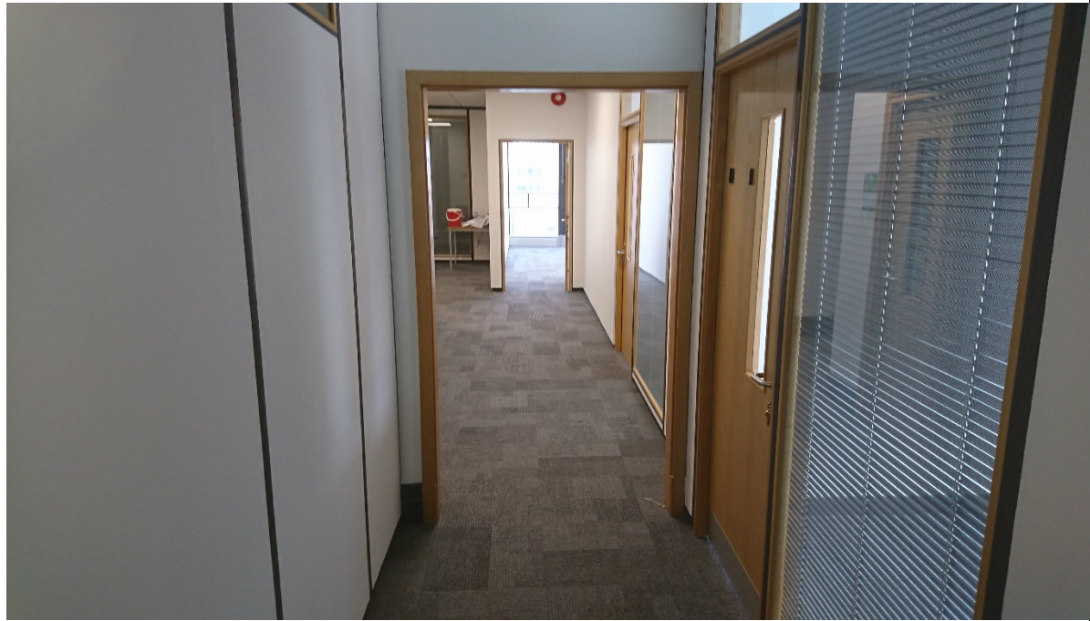
04-26 Looking north along a corridor with non-original partitioning and doors.
