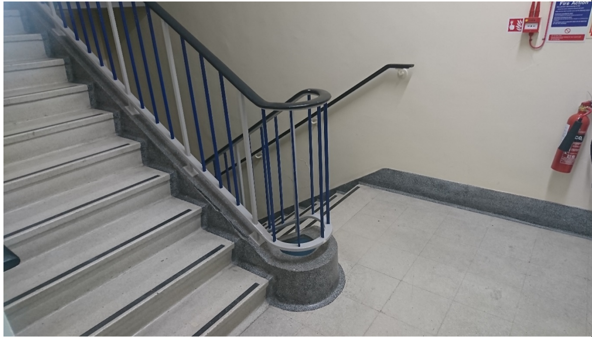
04-20 View within the eastern stair of the podium.
