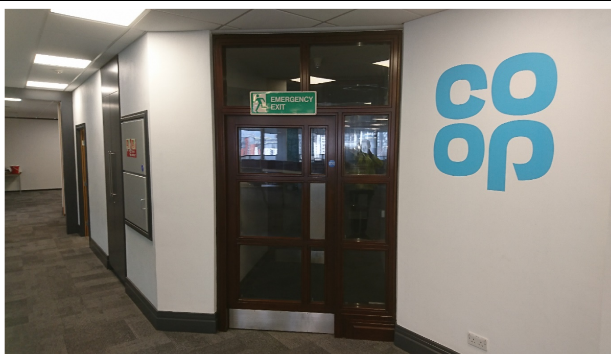
04-32 View of original doors that lead to the escalator.
