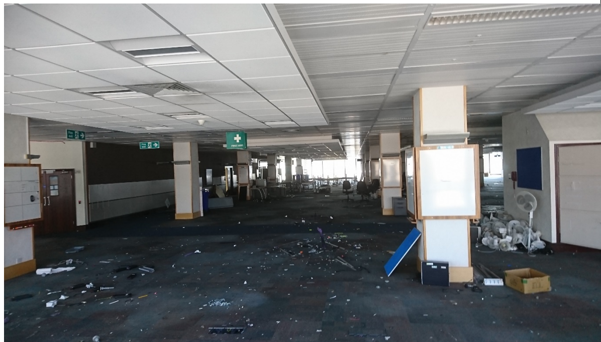
04-15 View across the open plan office from the west looking east.
