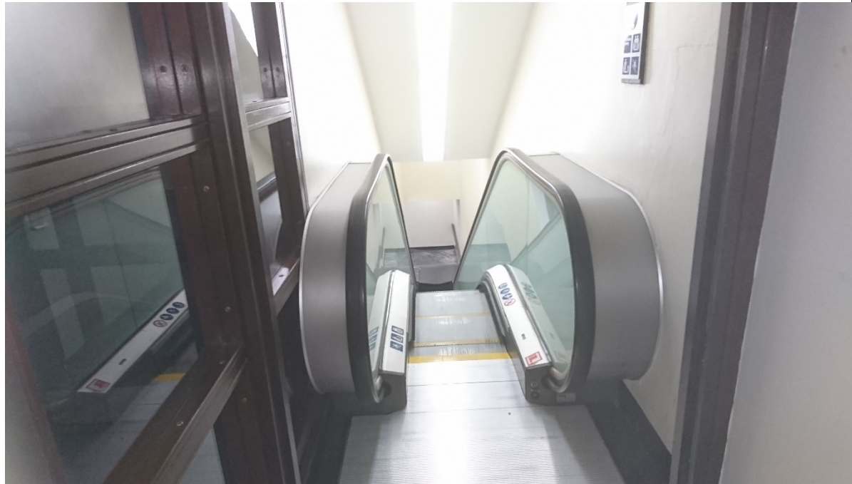
04-34 View looking down the escalator.
