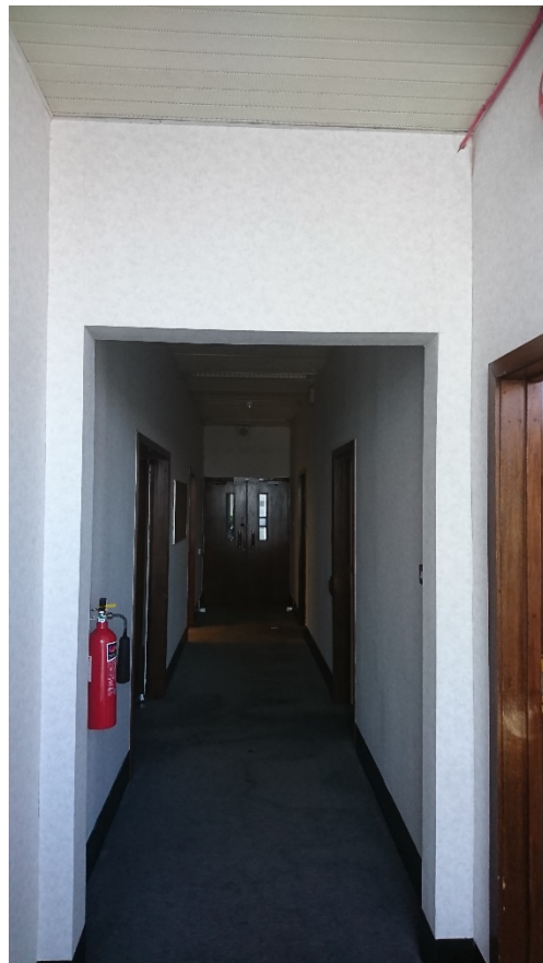
04-11 View down corridor with original door surviving.
