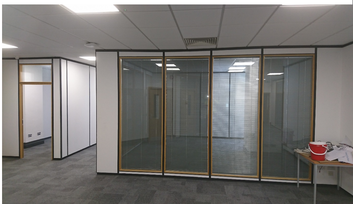
04-30 Typical view of office partitioning and ceilings.
