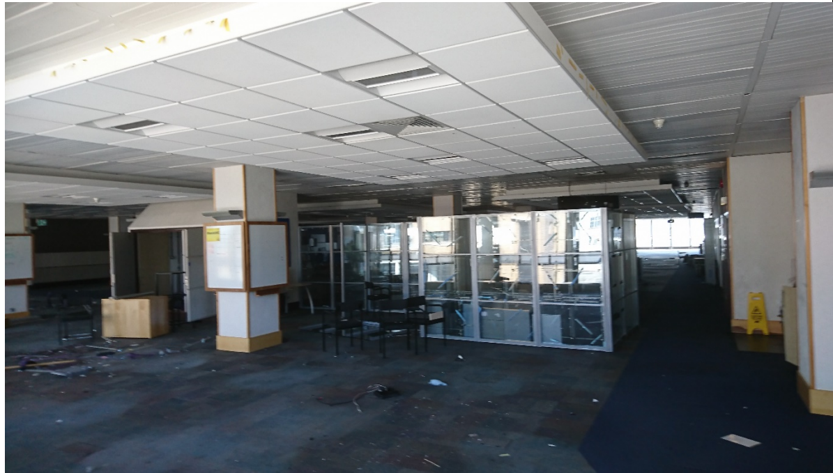
04-16 View of the Perspex partitioning to separate areas of the open plan office.
