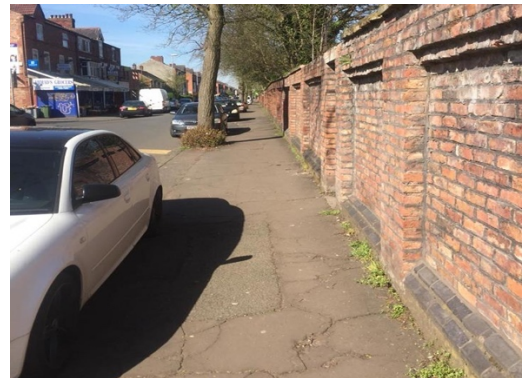
Footway on Clarendon Road
