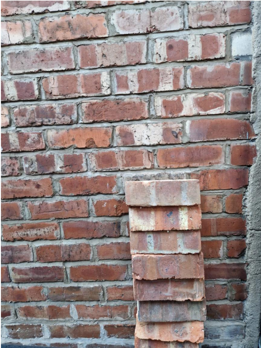
Photograph of proposed brickwork against the existing walls of the property.
