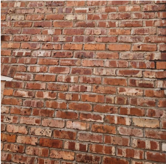
Photograph of existing brickwork of dwelling
