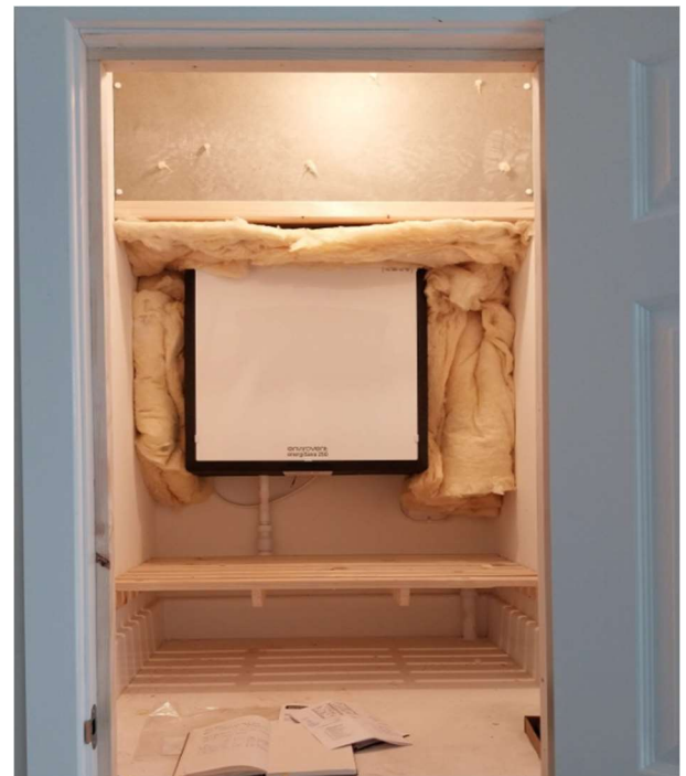
Figure 3-1: Plot 1 Mitigation measures
