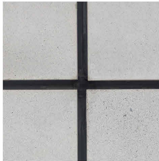
Existing Retained and Cleaned
