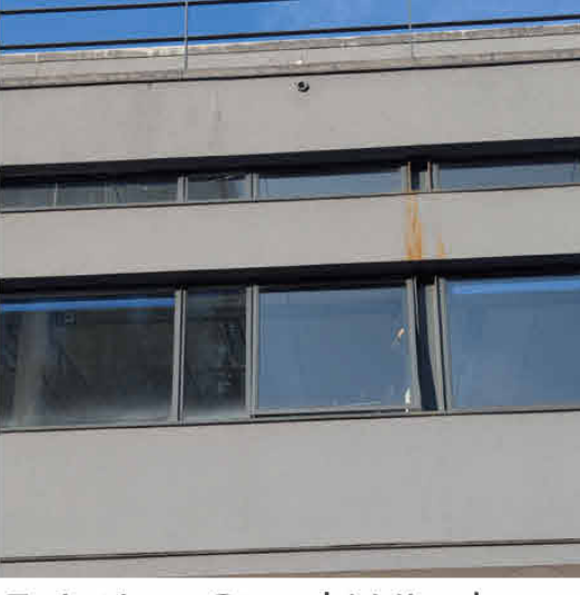
Existing Steel Window
