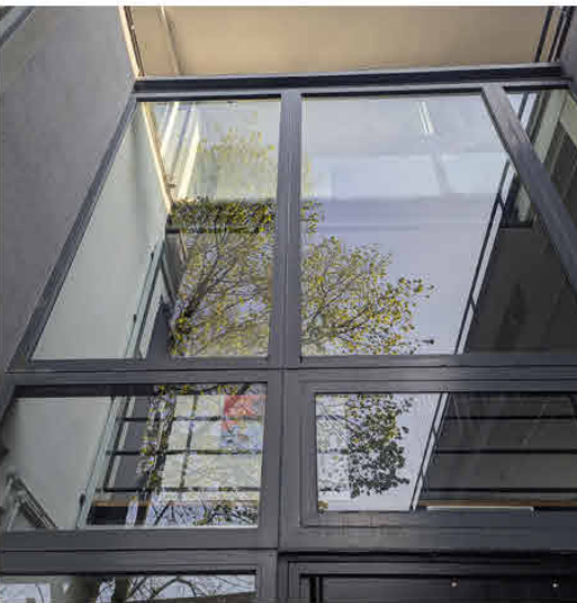
Existing Atrium Walling
