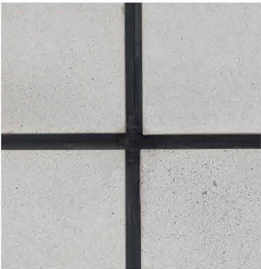
Existing Concrete Panel
