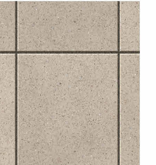
Existing Retained and Cleaned
