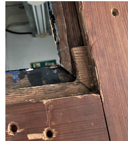
10mm thick panel example. Panel and one side of beading removed.
