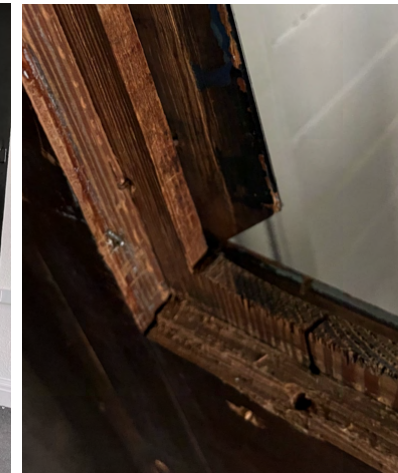
10mm thick panel example. Panel and one side of beading removed.
