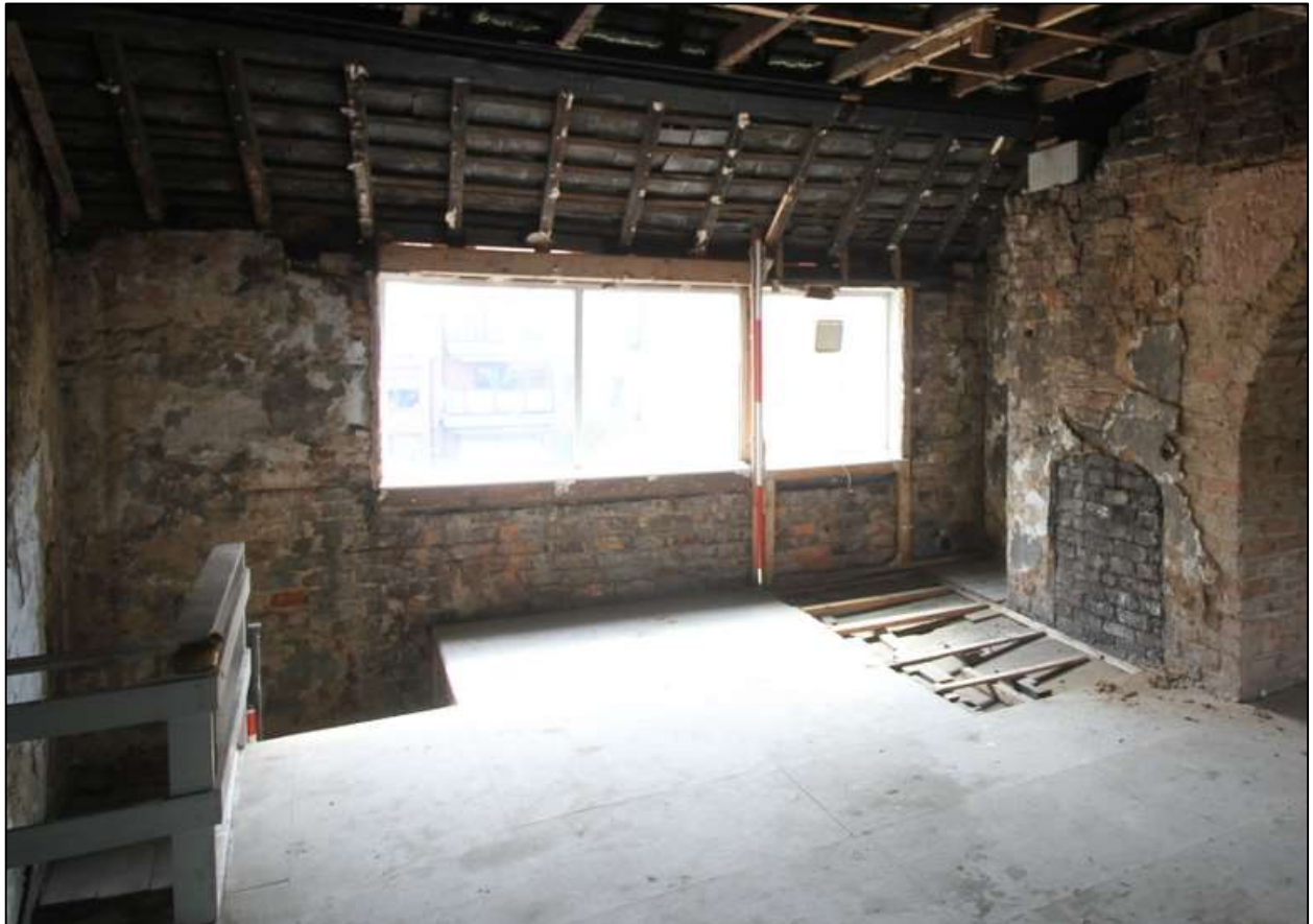
Plate 53: General view of the upper floor, looking south
