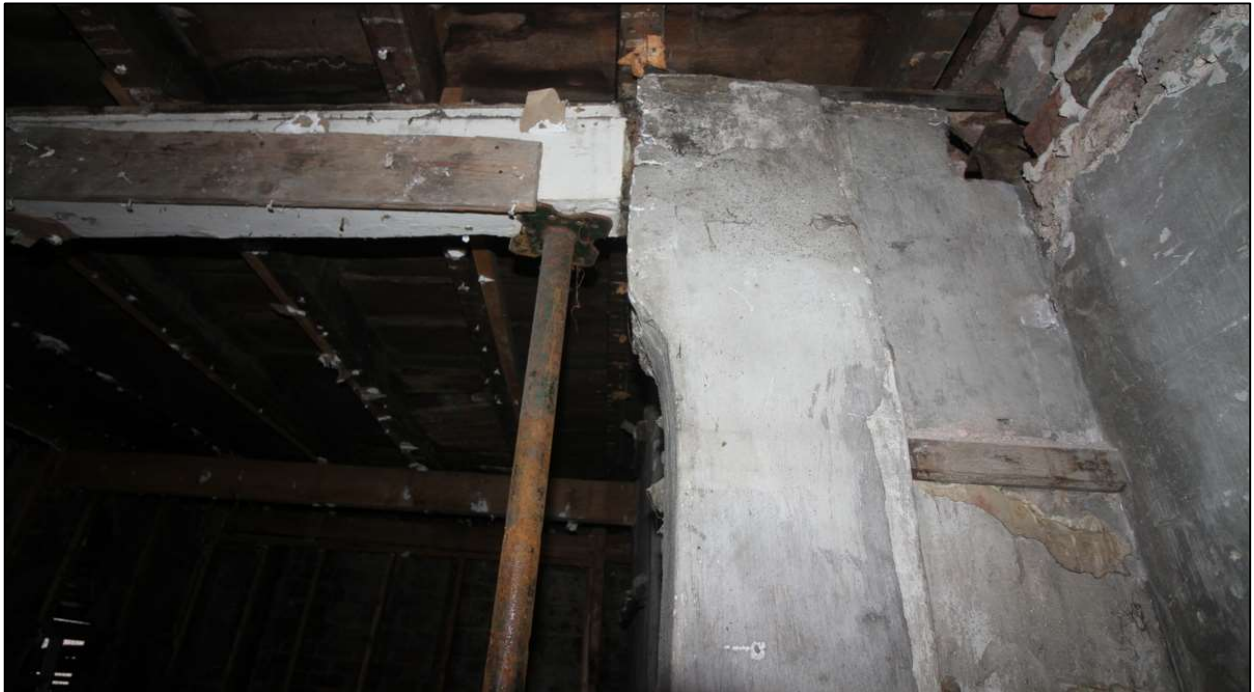
Plate 49: Detail of cross wall stub, with arched head
