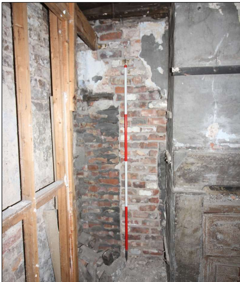
Plate 48: Blocked narrow doorway between 35 and 37 Liverpool Road
