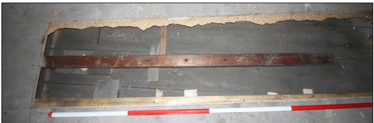
Plate 54: Detail of ladder rail used in floor levelling beneath the extant chipboard sheeting
