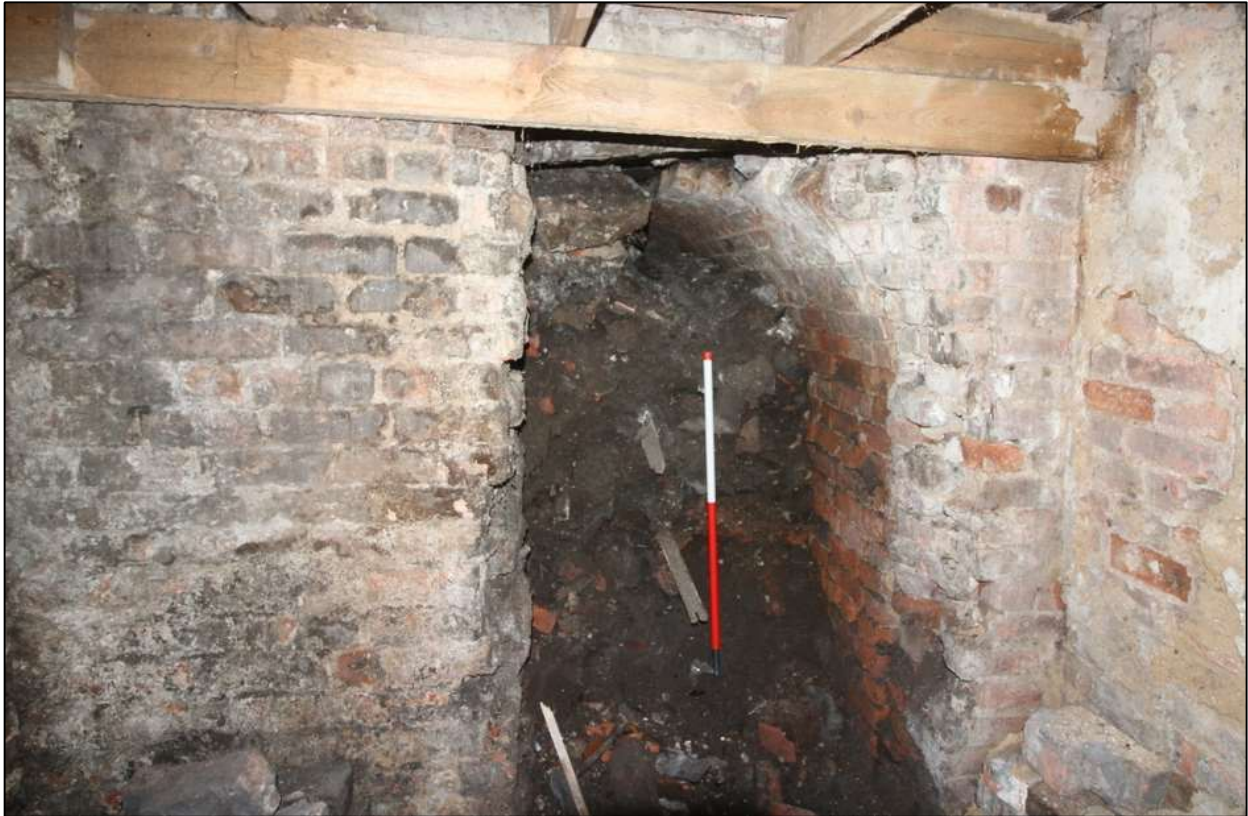
Plate 43: Vaulted chamber butted against the rear wall of the cellar
