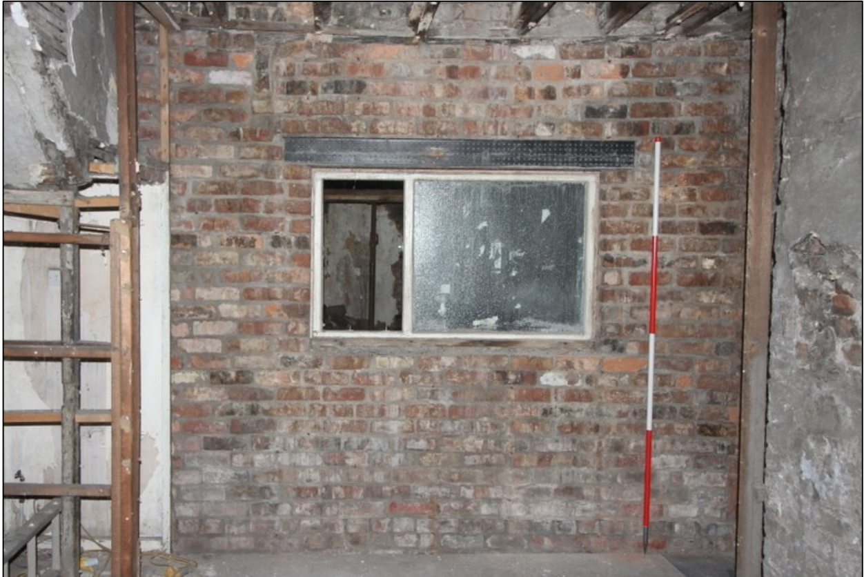
Plate 35: Rebuilt wall in position of original south external wall at ground floor level
