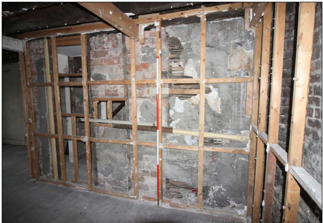
Plate 45: Partition wall to stair landing at first floor level
