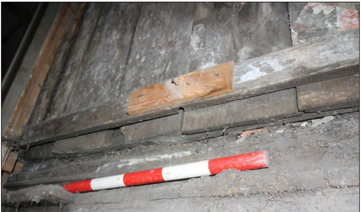
Plate 31: Detail of lap-jointing of timber planks on the inner face of the stair wall, with ends of planked floor boards below scale bar
