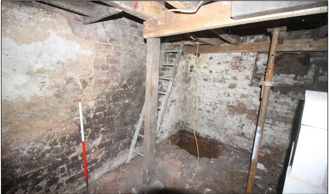
Plate 37: General view of the rear cellar, showing the extant ladder access to the ground floor
