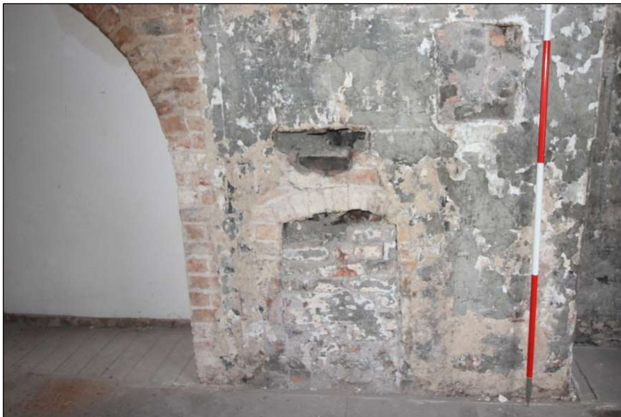
Plate 58: Detail of the northern fireplace in the west wall of the upper floor
