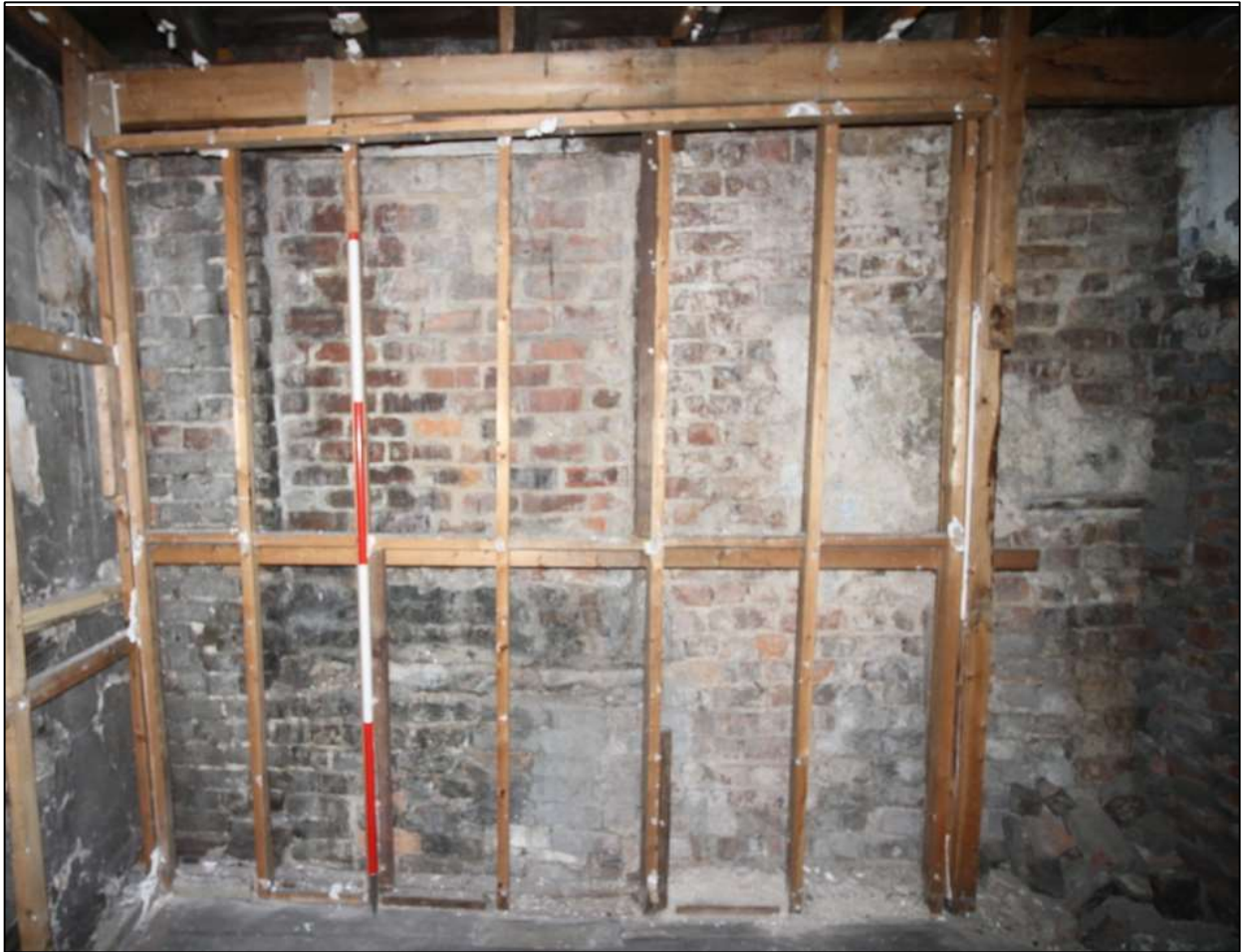
Plate 46: Timber studs from plasterboard wall concealing original rear wall with central brick-blocked window
