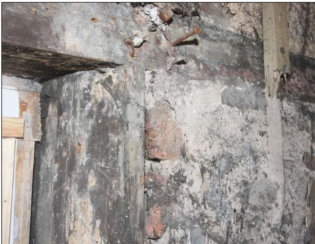
Plate 56: Detail of original chamfered window mullion head, below extant full-length lintel
