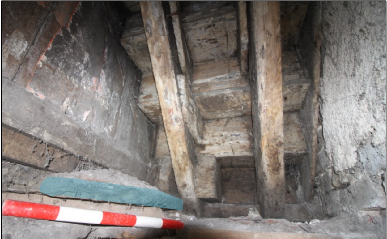
Plate 32: Underside of ground floor stairs, with planked partition and remnant of flagged floor (highlighted)
