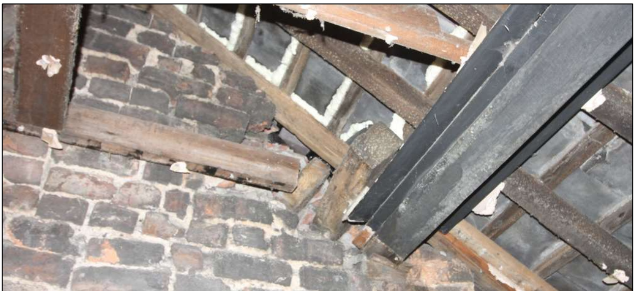
Plate 61: Purlin on south pitch projecting through wall from 33 Liverpool Road
