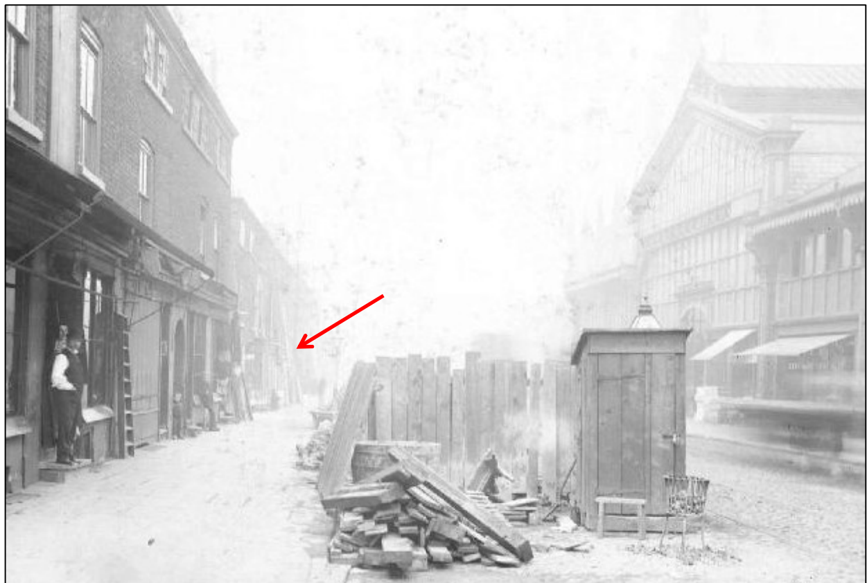
Plate 18: Contemporary, more oblique view of road repairs, showing ladders stacked outside Herbert Neild's premises at 21 Liverpool Road (highlighted) ©Manchester Libraries
