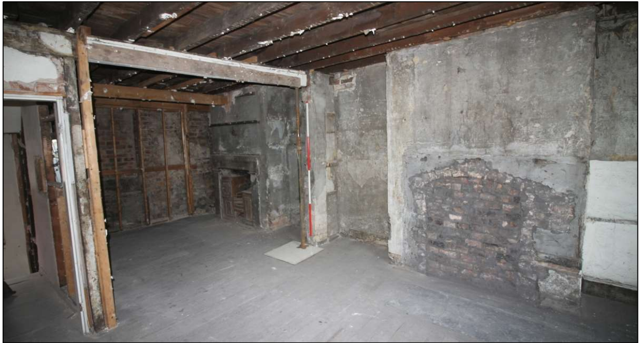
Plate 44: General view of the first floor, looking south-west
