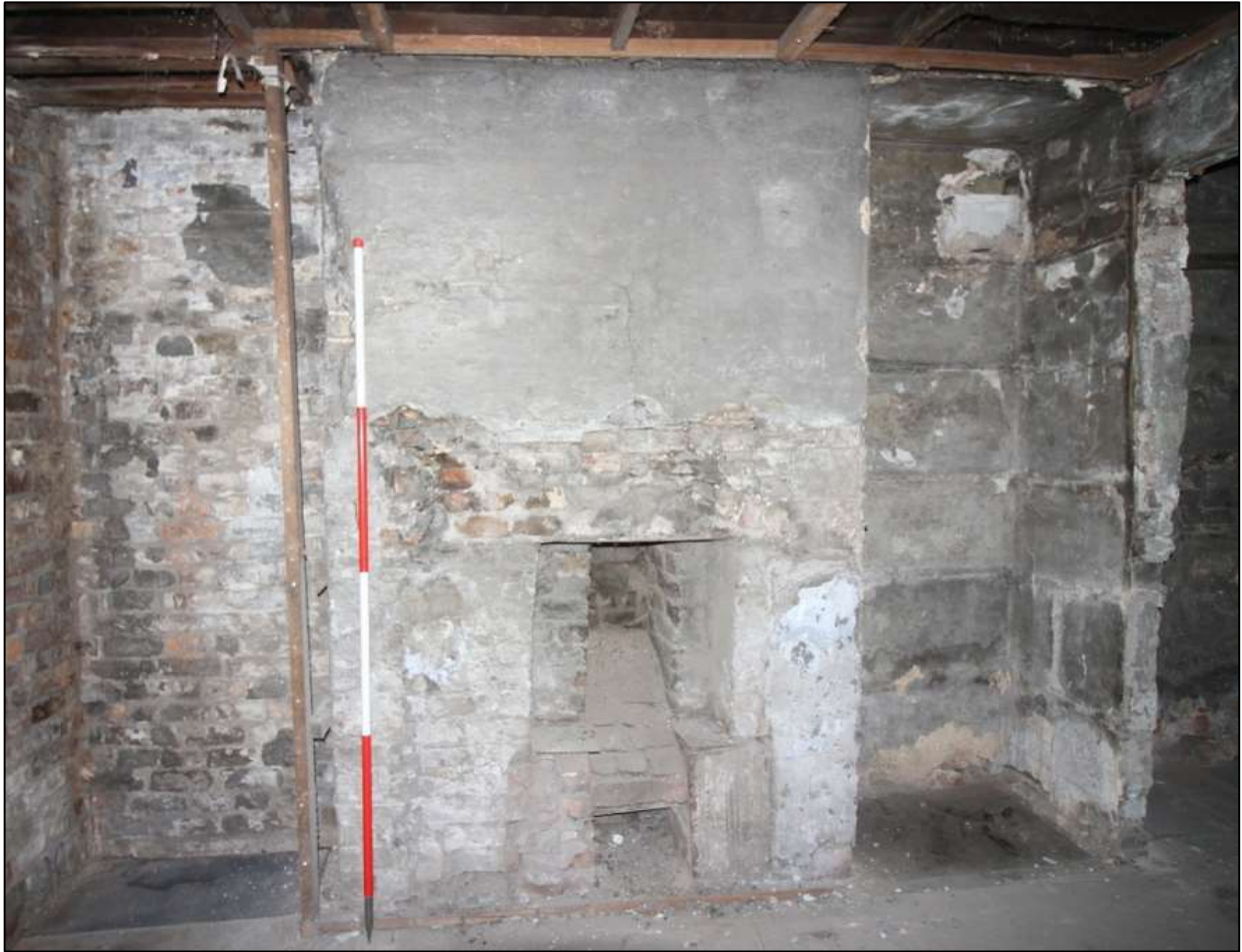
Plate 29: Fireplace in rear room of ground floor with cast iron framing and stub of original partition (right)
