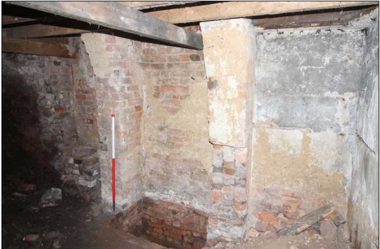
Plate 41: Brick piers for ground-floor level chimney breast and hearth stone in rear room of cellar
