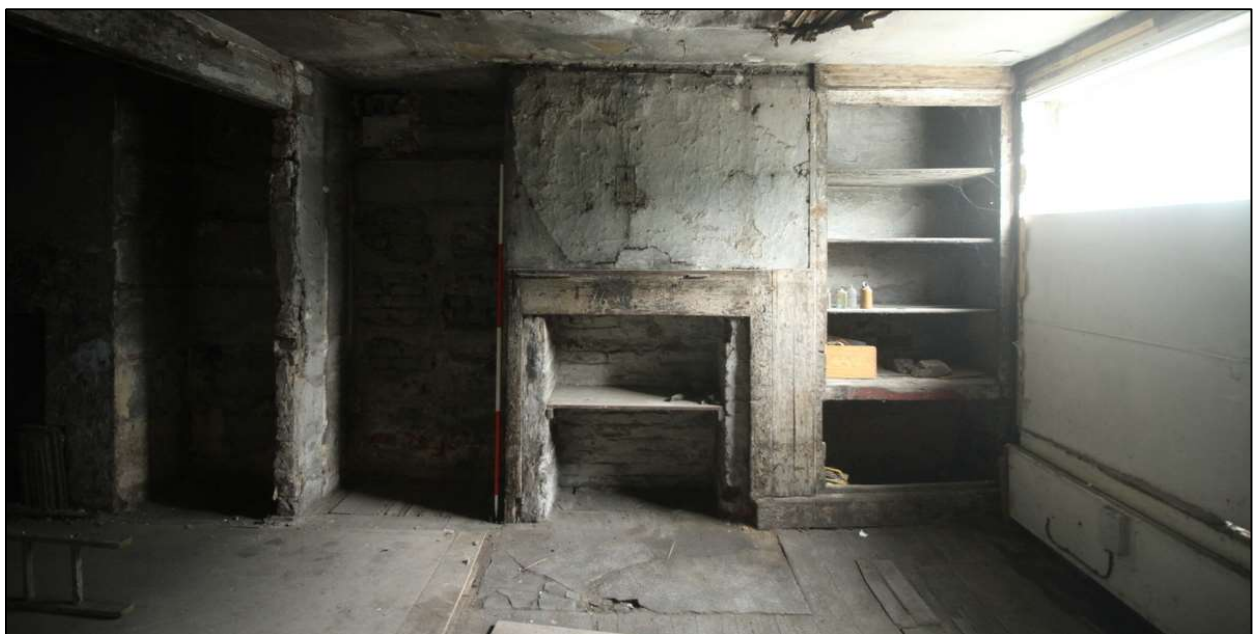
Plate 28: Fireplace in northern 'front' room of ground floor with hearthstone and shelved alcove
