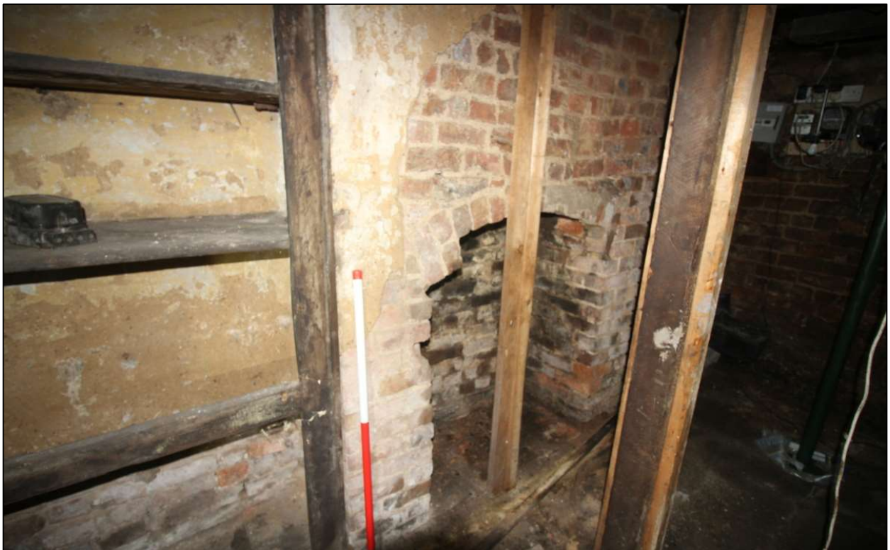
Plate 39: Fireplace in west wall of northern cellar room, with later shelving to alcove
