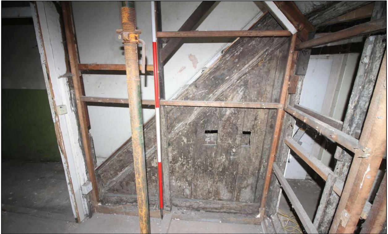
Plate 30: Timber-planked stair wall revealed by the removal of late stud partitioning
