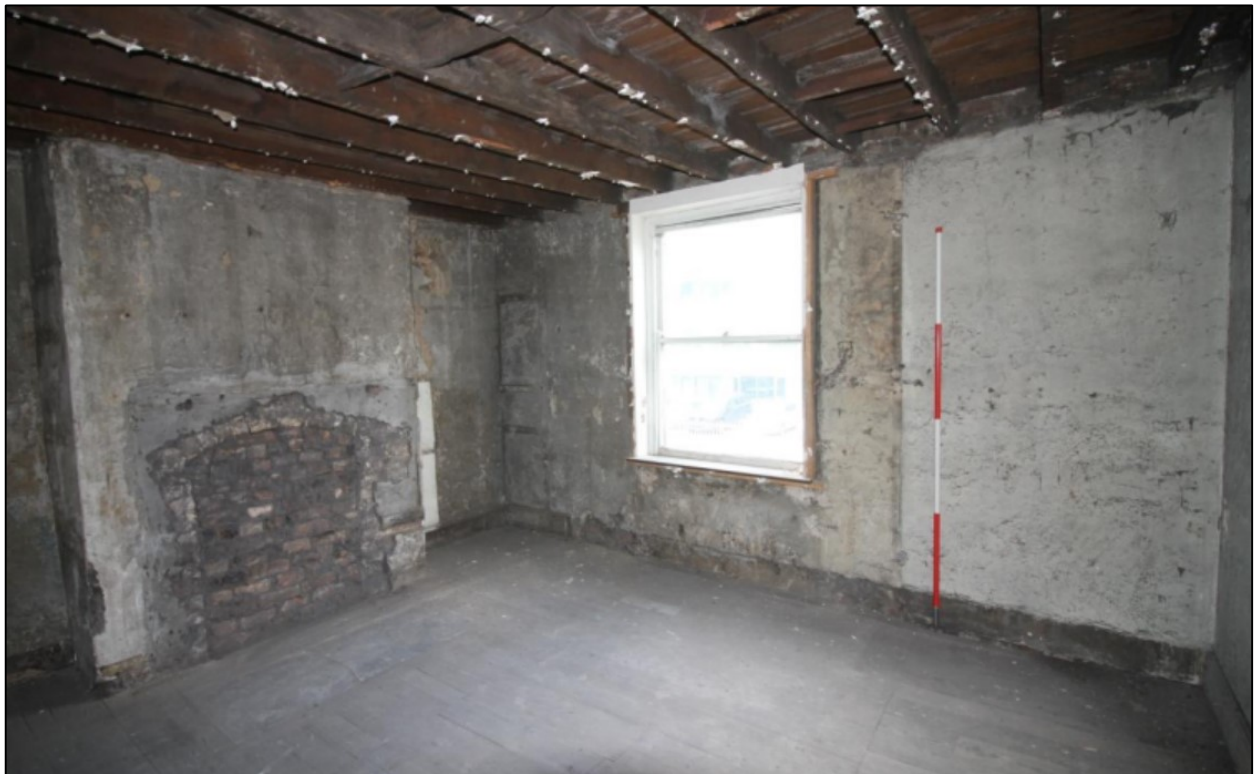
Plate 50: North room at first-floor level
