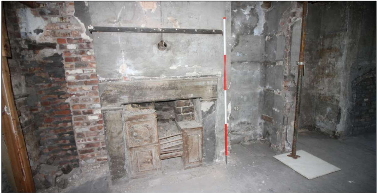
Plate 47: detail of fireplace in the rear room at first-floor level, with ladder rail mounted above
