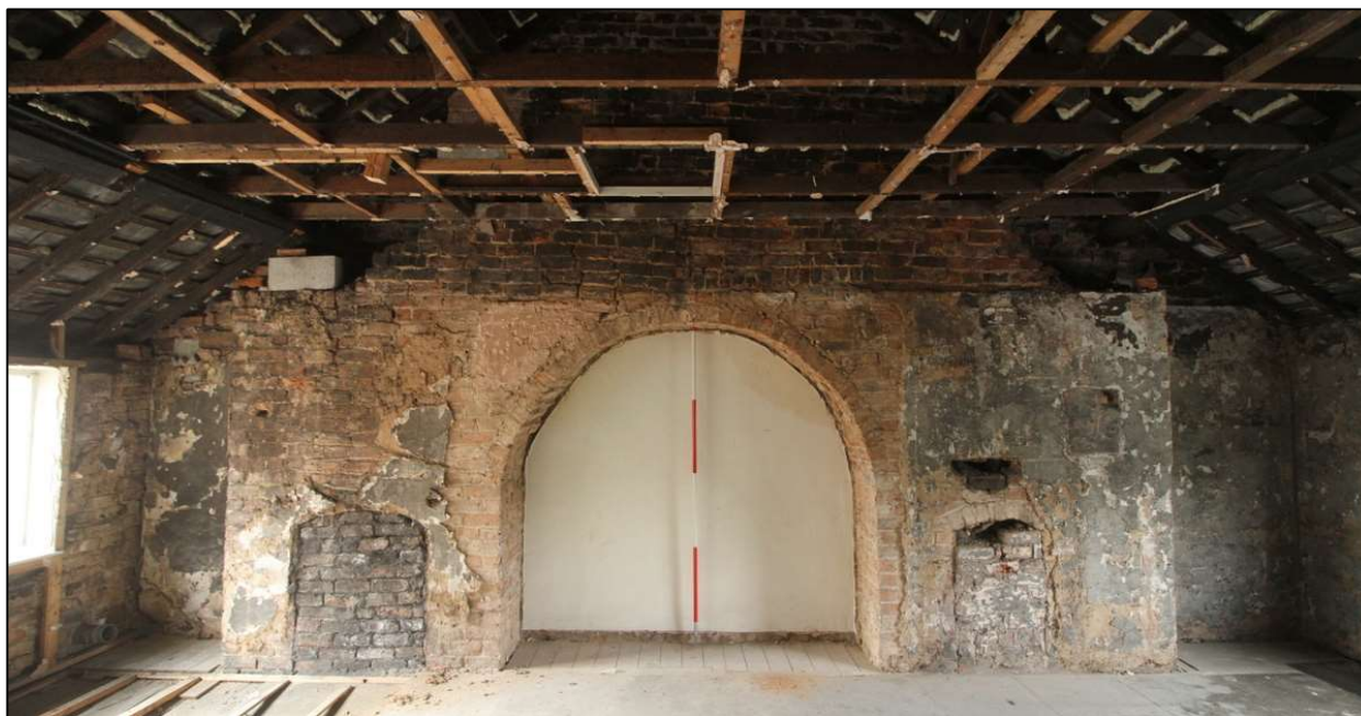
Plate 57: Fireplaces and flues against the west wall of the upper floor
