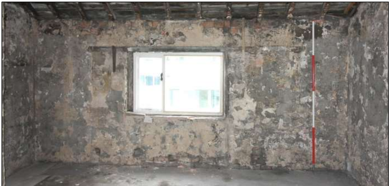
Plate 55: Narrowed garret window in north wall, retaining lintel across the original wider aperture
