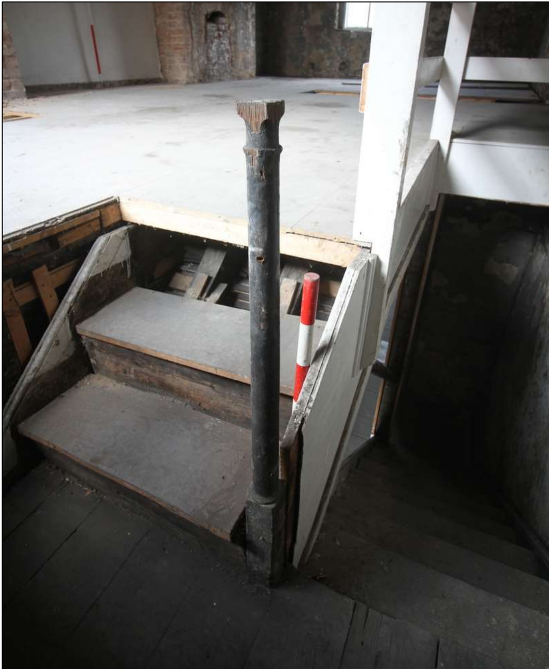
Plate 52: Detail of half-landing and possibly original newel post to the upper floor stair
