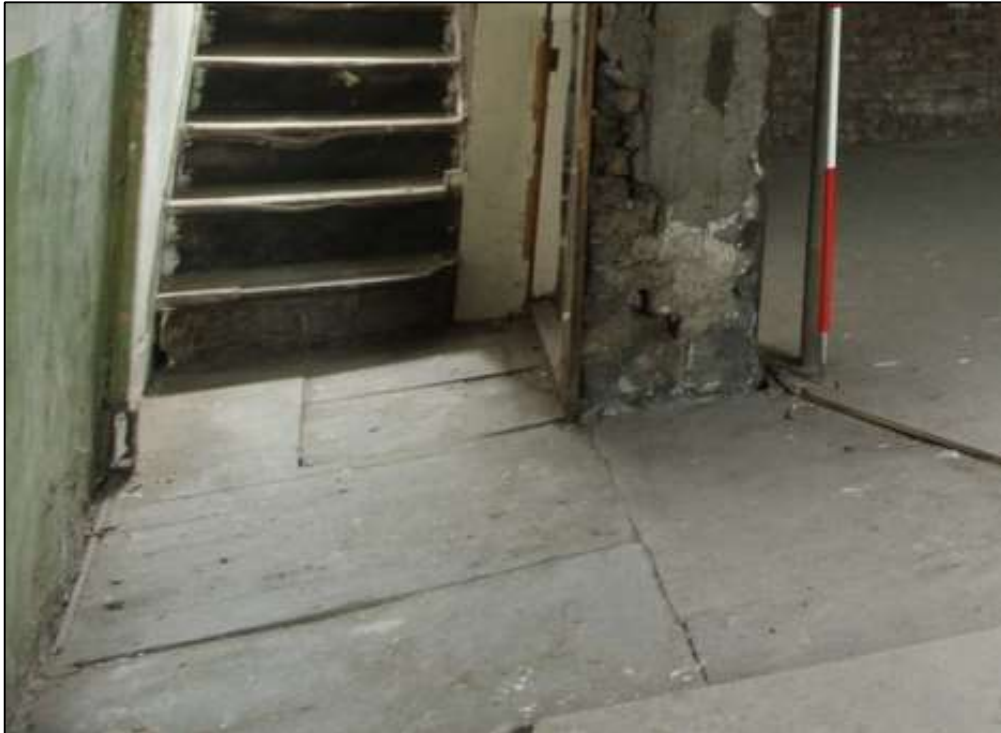
Plate 33: Flagstones set within planked corridor at foot of the stairs to first floor
