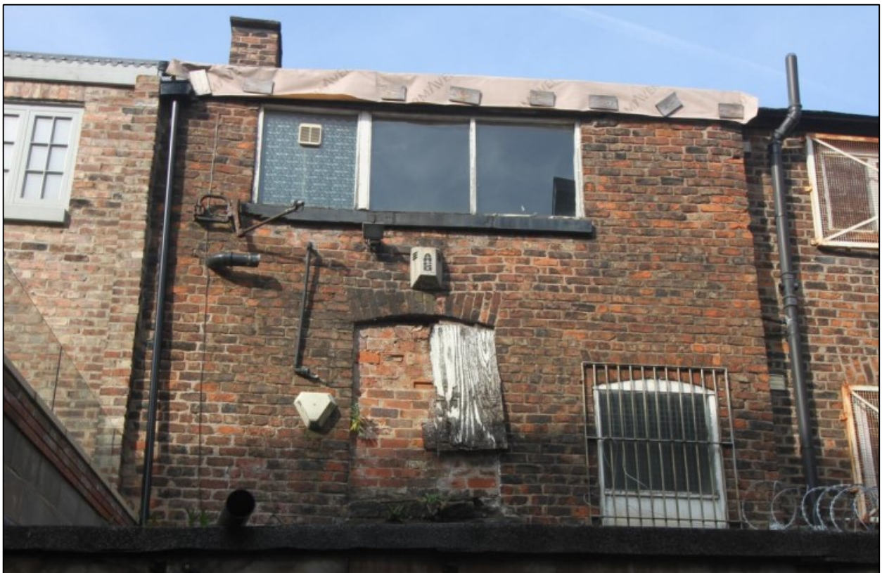
Plate 26: Rear of 35 Liverpool Road, above the late single-storey extension, showing no wall scars for a 'back extension'
