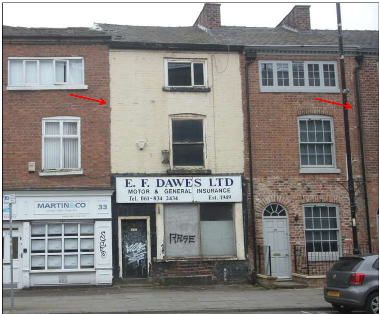
Plate 24: Principal façade of 35 Liverpool Road (painted in the late 20 th century) with vertical construction breaks to 33 and 39 Liverpool Road (highlighted)
