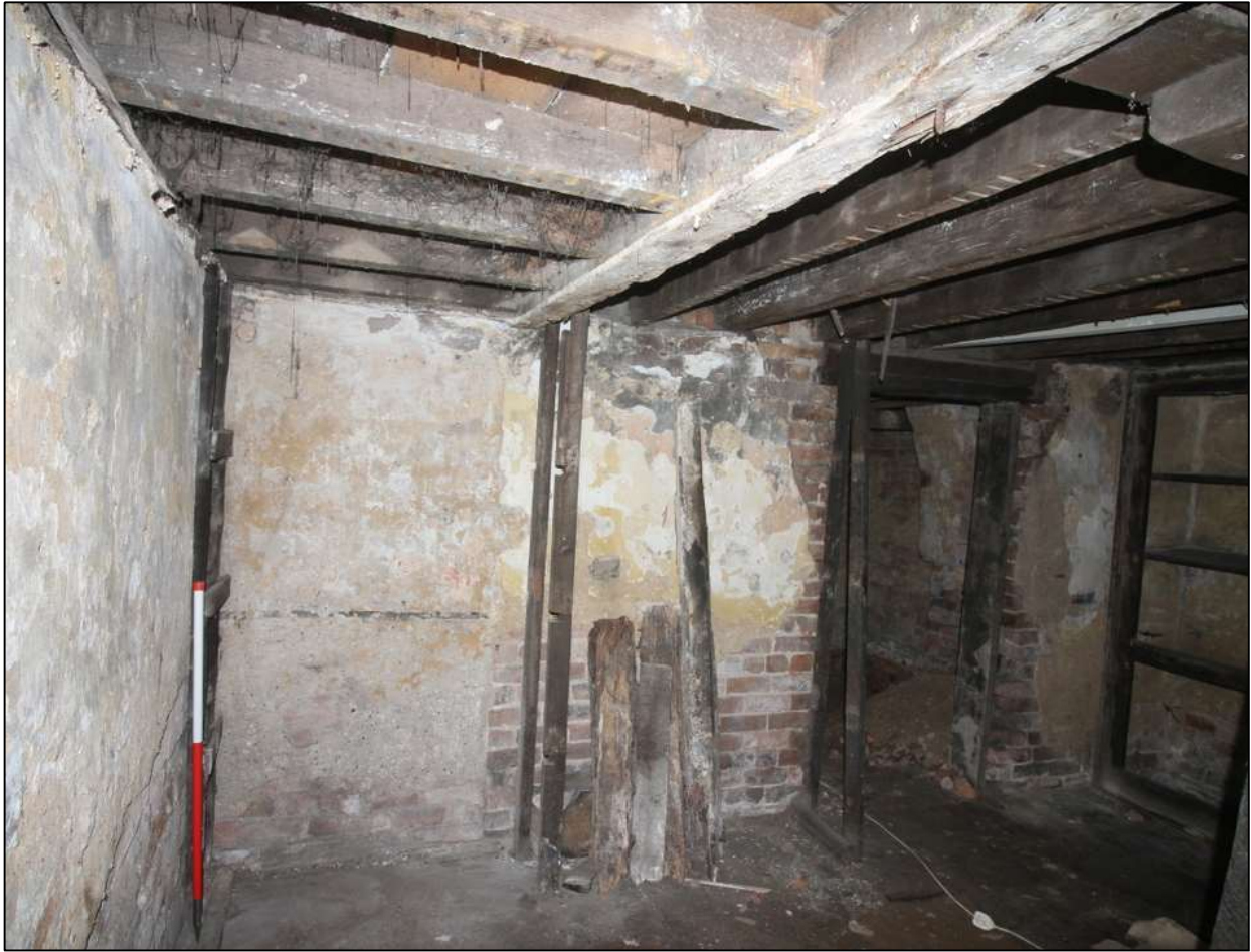
Plate 40: Differing arrangement of ceiling joists in cellar suggesting passage to blocked doorway in partition wall, with later doorway inserted to right
