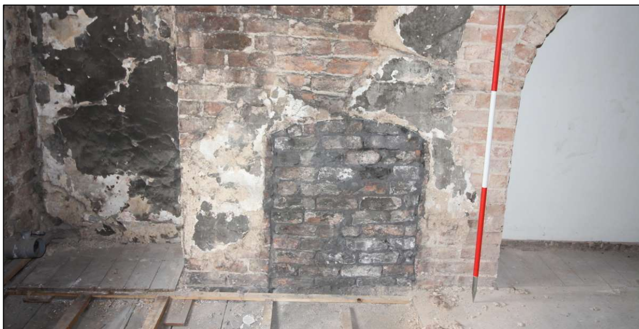
Plate 59: Detail of the southern fireplace in the west wall of the upper floor
