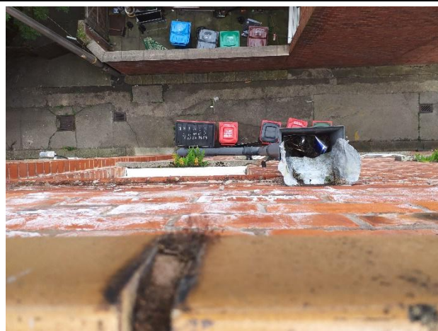
Image 76: Debris in rainwater hoppers at rear.
