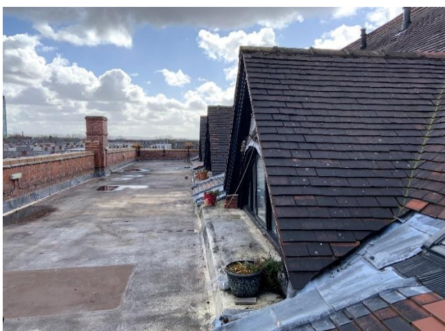
View of rear flat roof and pitched roof
