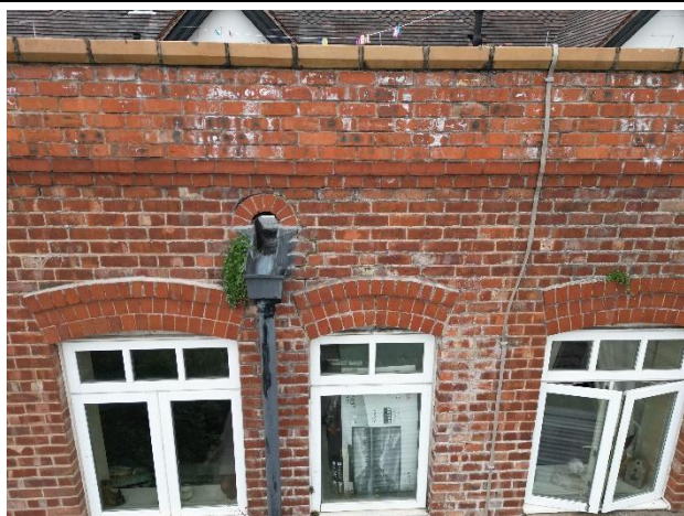
Image 75: Degraded masonry jointing & minor decay to rear elevation windows.
