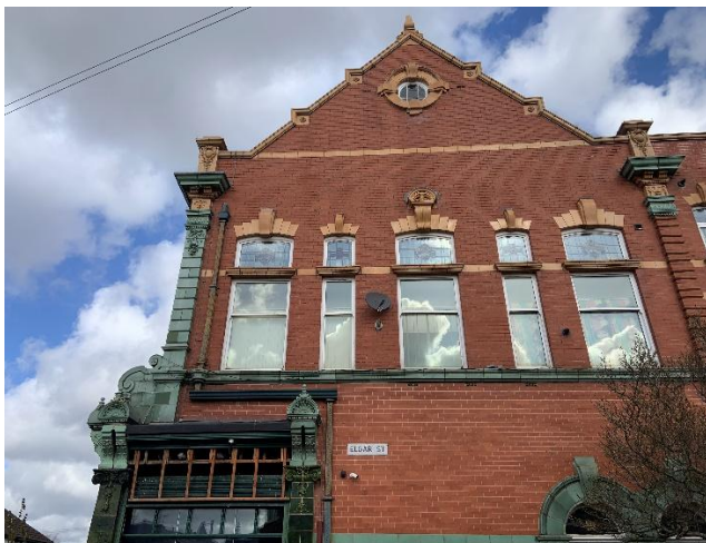
View of South Elevation – Elgar Street
