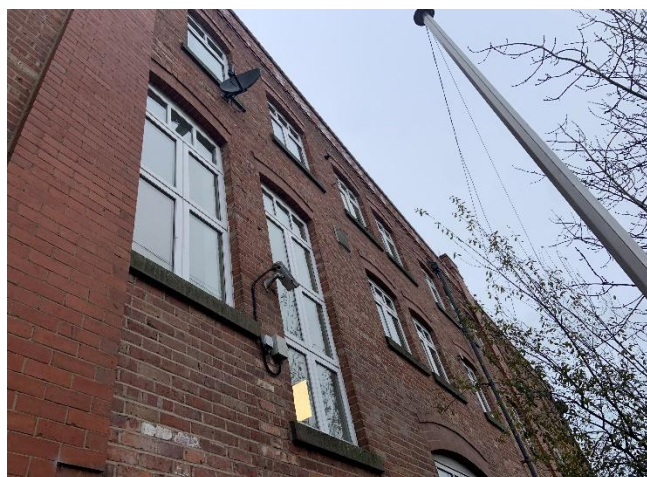
View of Rear Elevation
