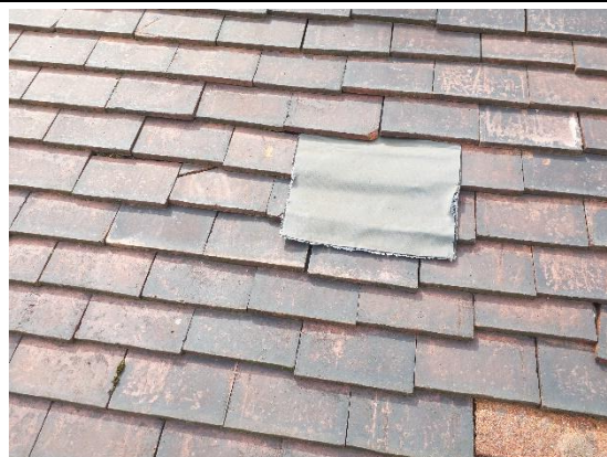
Image 78: Poor quality repairs to tile coverings.
