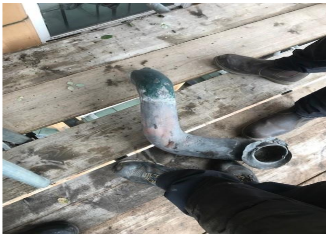
Image 73: Investigations to front elevation revealed, section of lead pipe required renewal.
