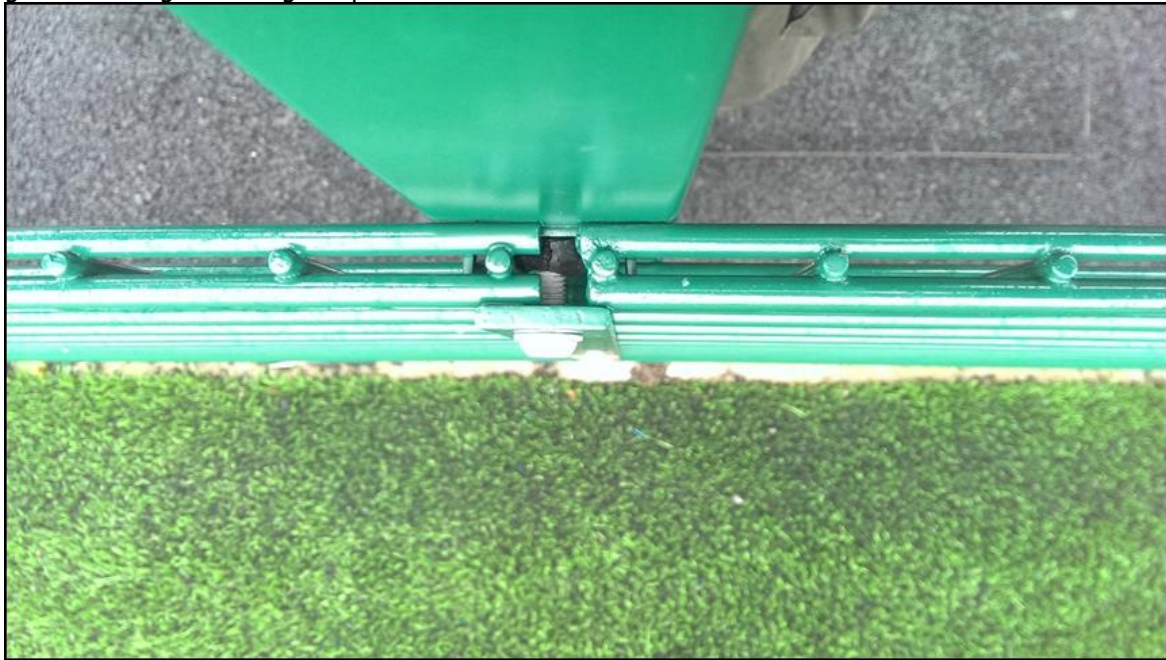
Figure 12: Image Showing Neoprene Isolators
