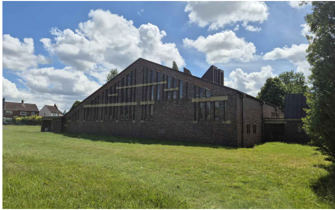
View from North-East
