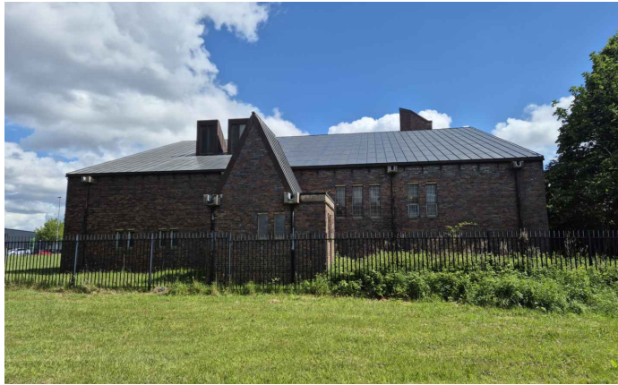
View from South-West
