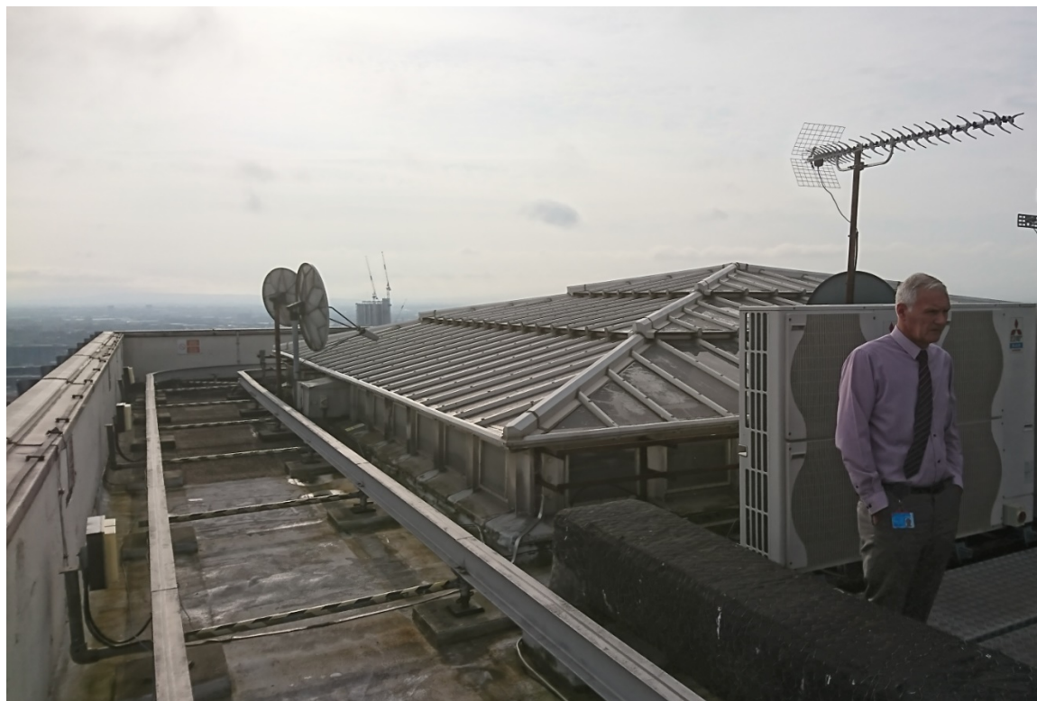
RL-03 Looking south-east from the parapet showing the track-bed for the window access plant and glazed pyramid roof lighting the east-side of level 25 below.
