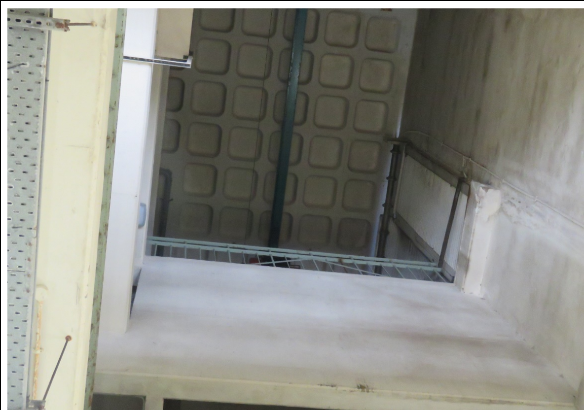
RL-08 Looking up the service tower to the coffered concrete roof above the lift overrun.
