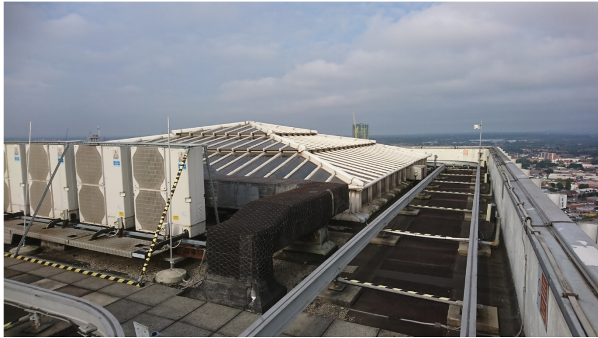
RL-02 Looking south-west from the parapet showing the track-bed for the window access plant and glazed pyramid roof lighting the west-side of level 25 below.
