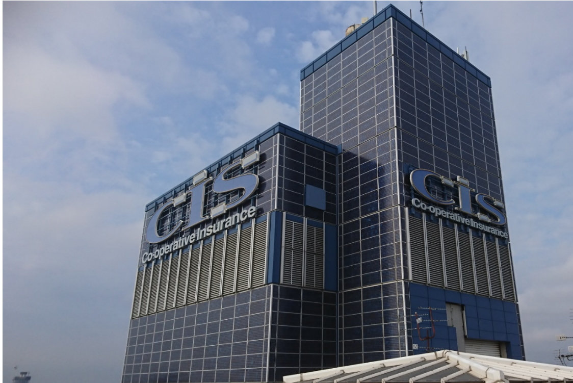
RL-06 Looking south-west from the south-east corner at the detail of the cladding of the service tower and signage.
