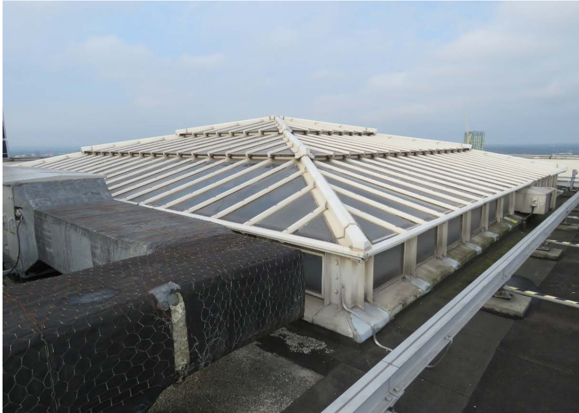
RL-04 Looking north from the south parapet showing detail of the structure of the glazed pyramid roof.
