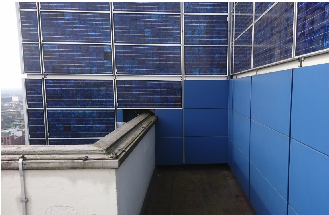
RL-07 Looking south showing the detail of the parapet, lightning conductor, photovoltaic panels and lower level cladding.
