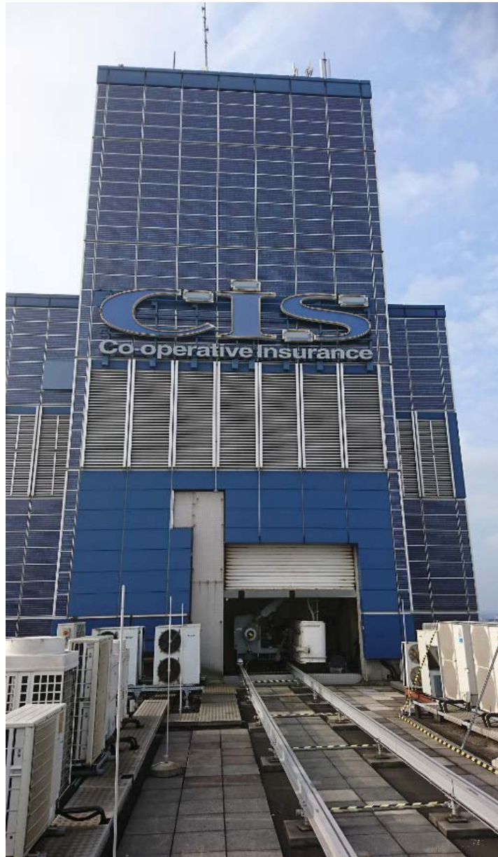
RL-01 Looking south from the parapet, showing the details of the applied signage and photovoltaic cells as well as the track access to the lift tower.
