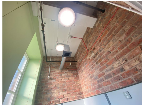
Example of WC Ceiling
