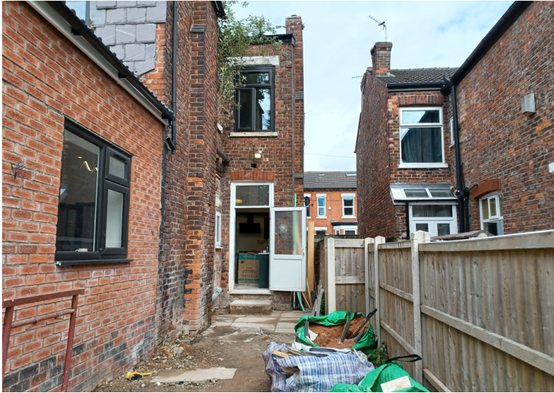
View of southern side elevation of rear extension
