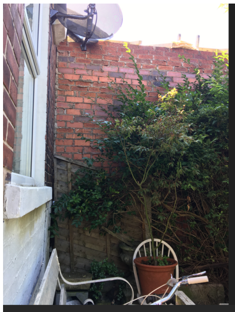
Views of partially built northern elevation of extension
