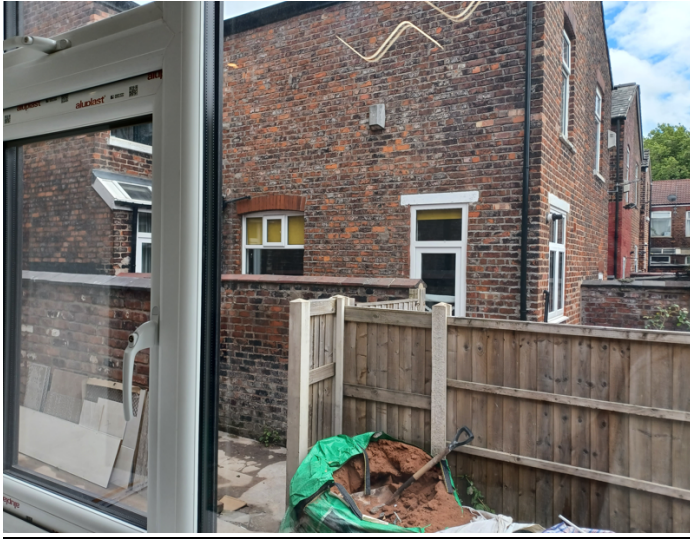
Views from the as built extension looking south
