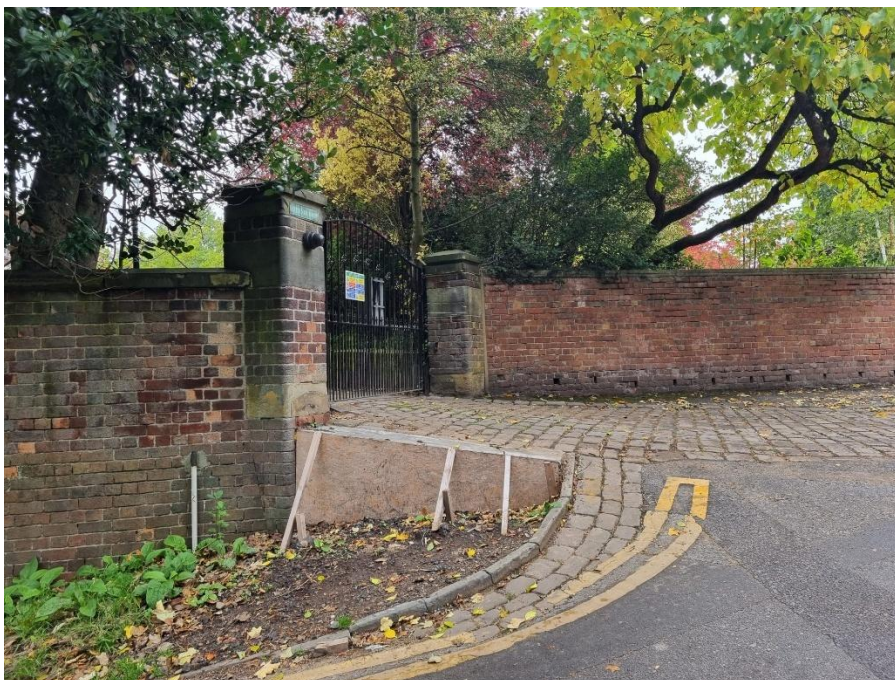
View of access gates to Stenner Brow from Stenner Lane
