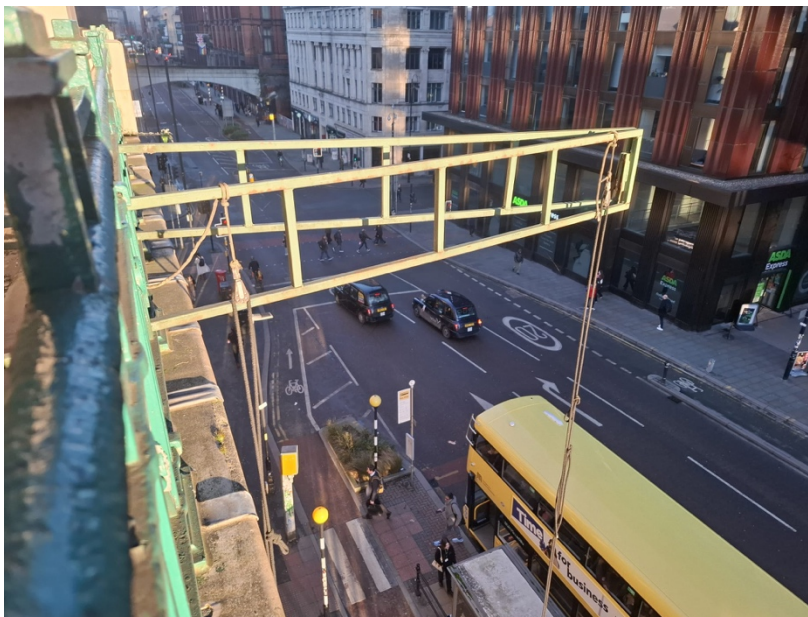
EXISTING BANNER GANTRY AND RIGGING ROPES
