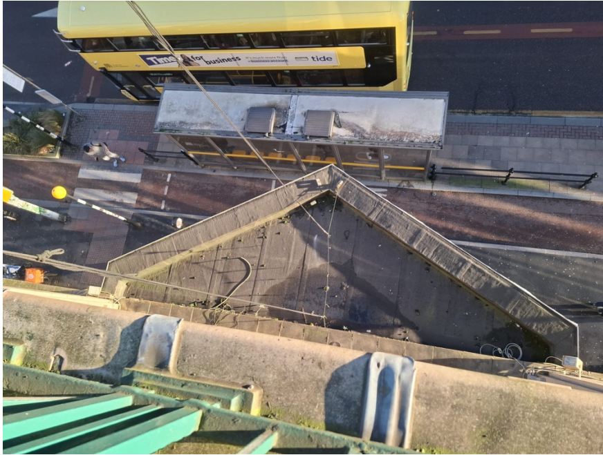
EXISTING CANOPY ROOF, BANNER RIGGING ROPES & TETHERS
