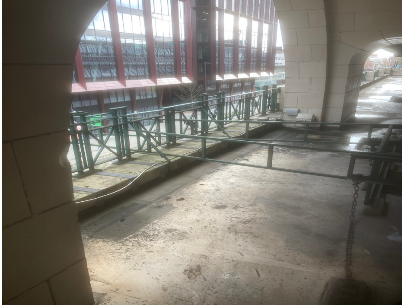
EXISTING BANNER GANTRY AT SECOND FLOOR LEVE
