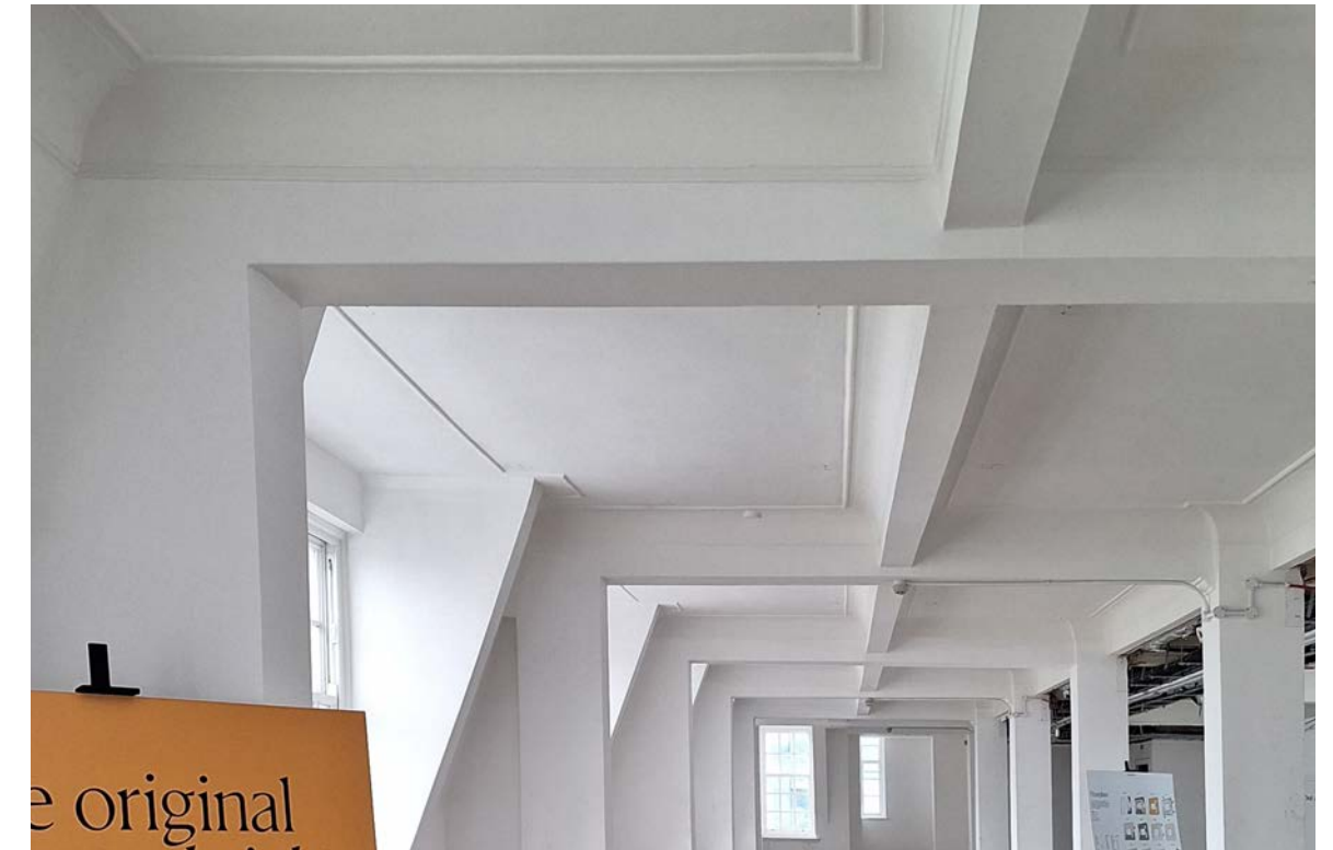
02 Existing coffered ceiling on Level 10
