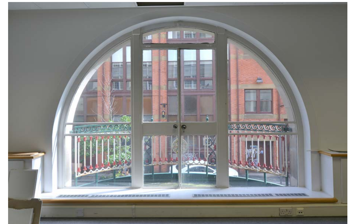
04 Arched window on Level 01
