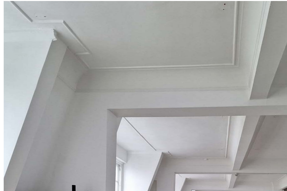
Existing coffered ceiling on Level 11
