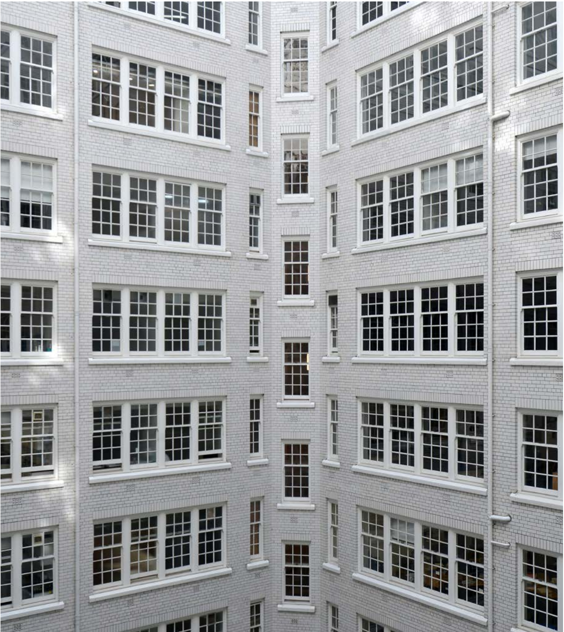
03 View of the internal atrium windows
