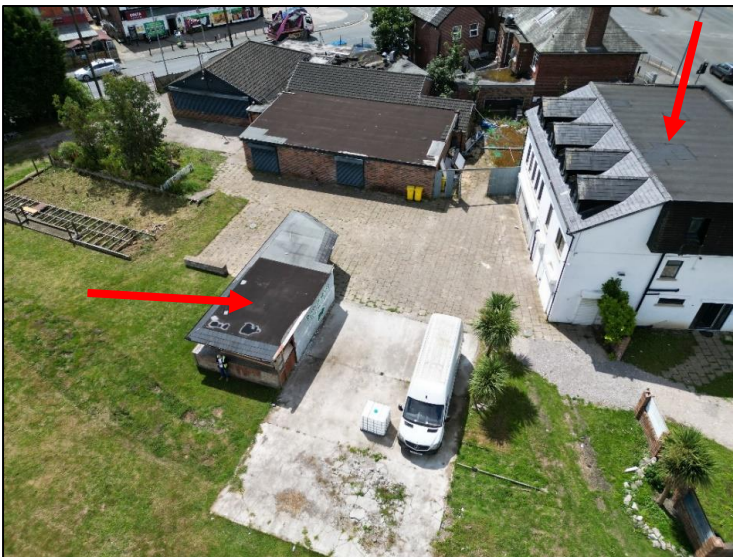
Photograph 4 showing B1 (on right) and B2 (on left)
