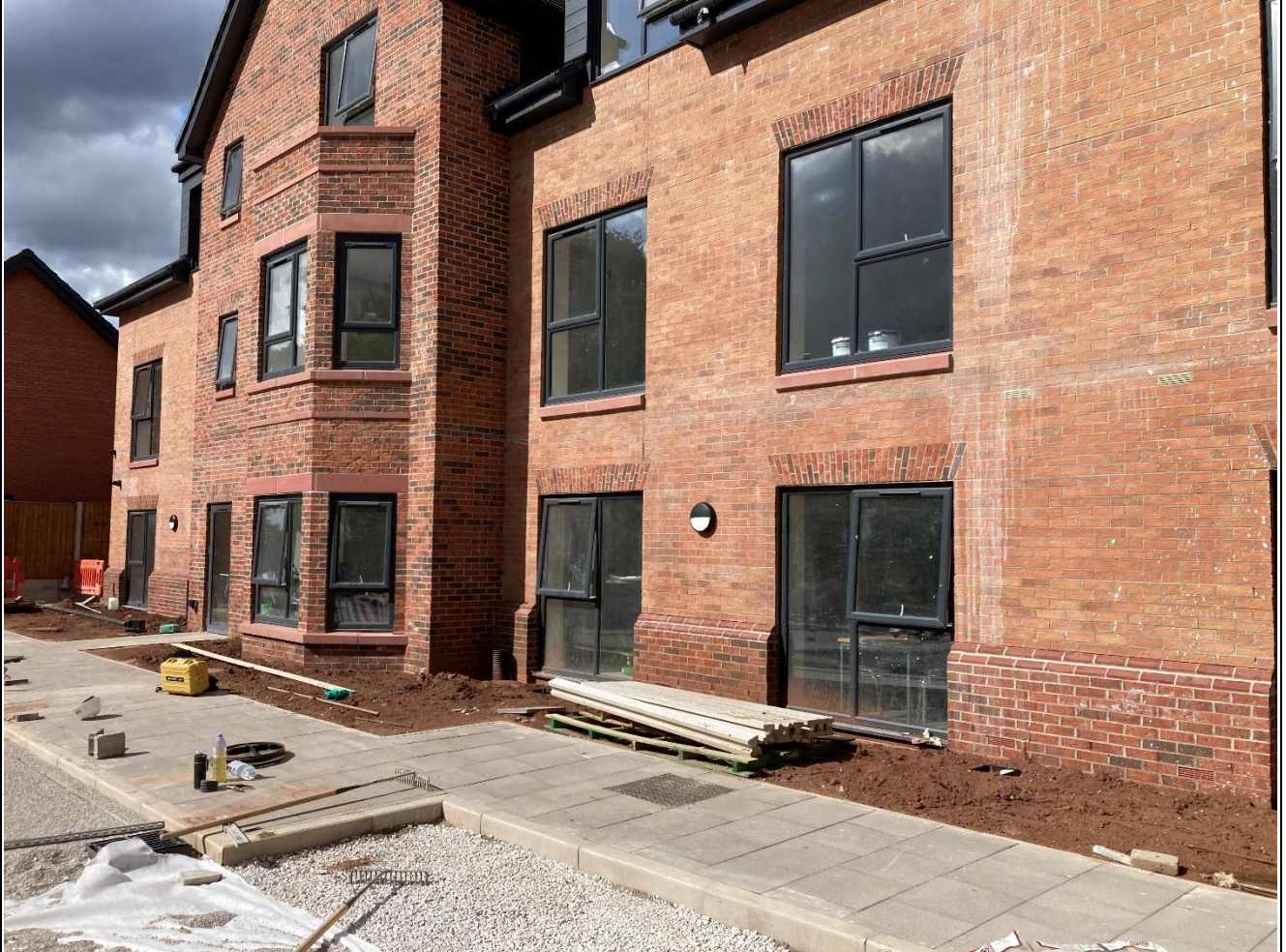
Figure 1: Front of building facing the car park, showing completed clean cover system. Facing northwest.
