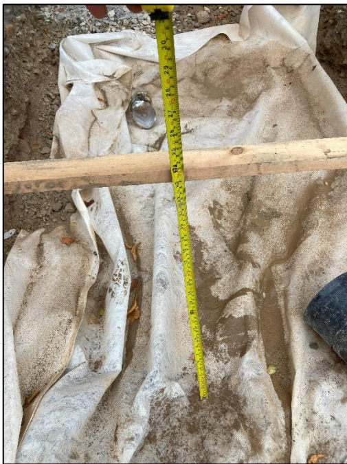
Reduced level dig and placement of membrane in rear garden (detail)
