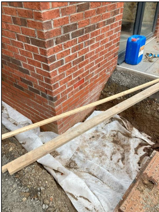
Geotextile placement, at a reduced level of 600mm
