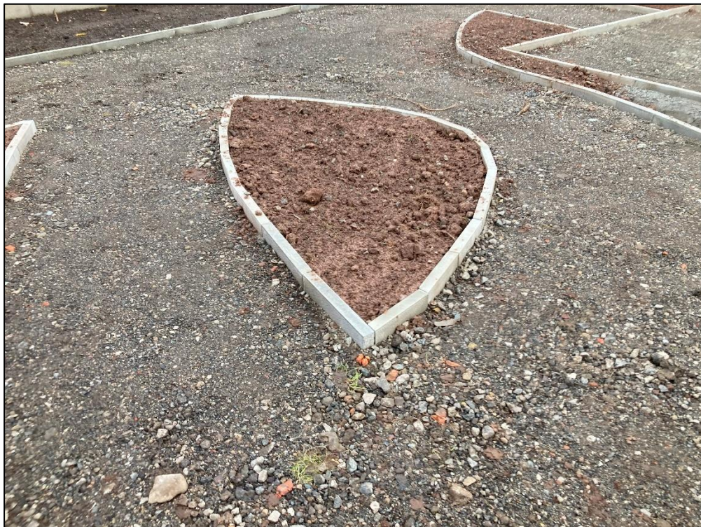
Soil being placed in rear landscaping areas adjacent to building
