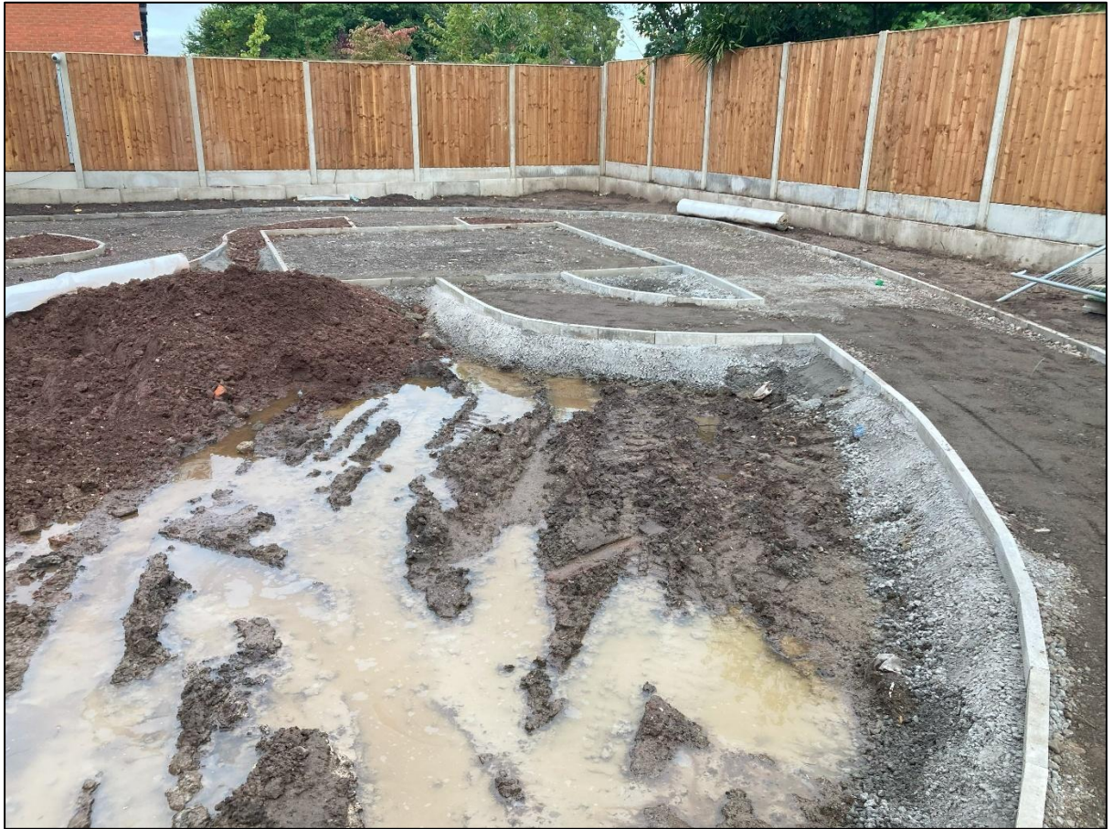
Path network being laid, soft landscaping areas in progress with reduced dig evident.
