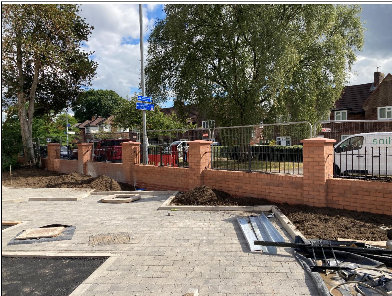
Figure 2: Southeastern area of the carpark, showing completed clean cover system. Facing southeast.
