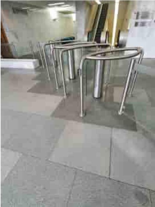
Patched floor under turnstiles
