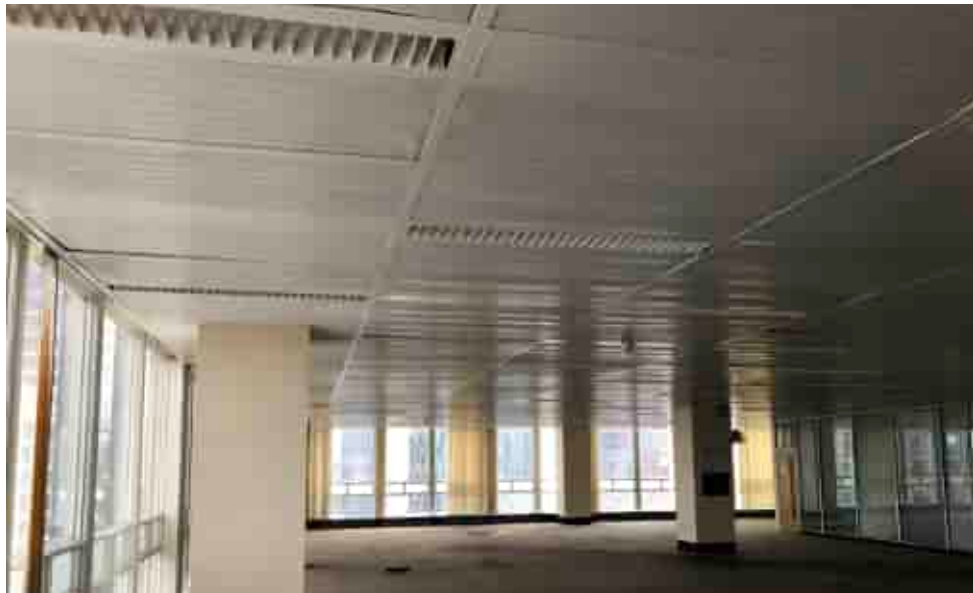
Existing ceiling integrating retrofitted, but aging, lighting and servicing grilles
