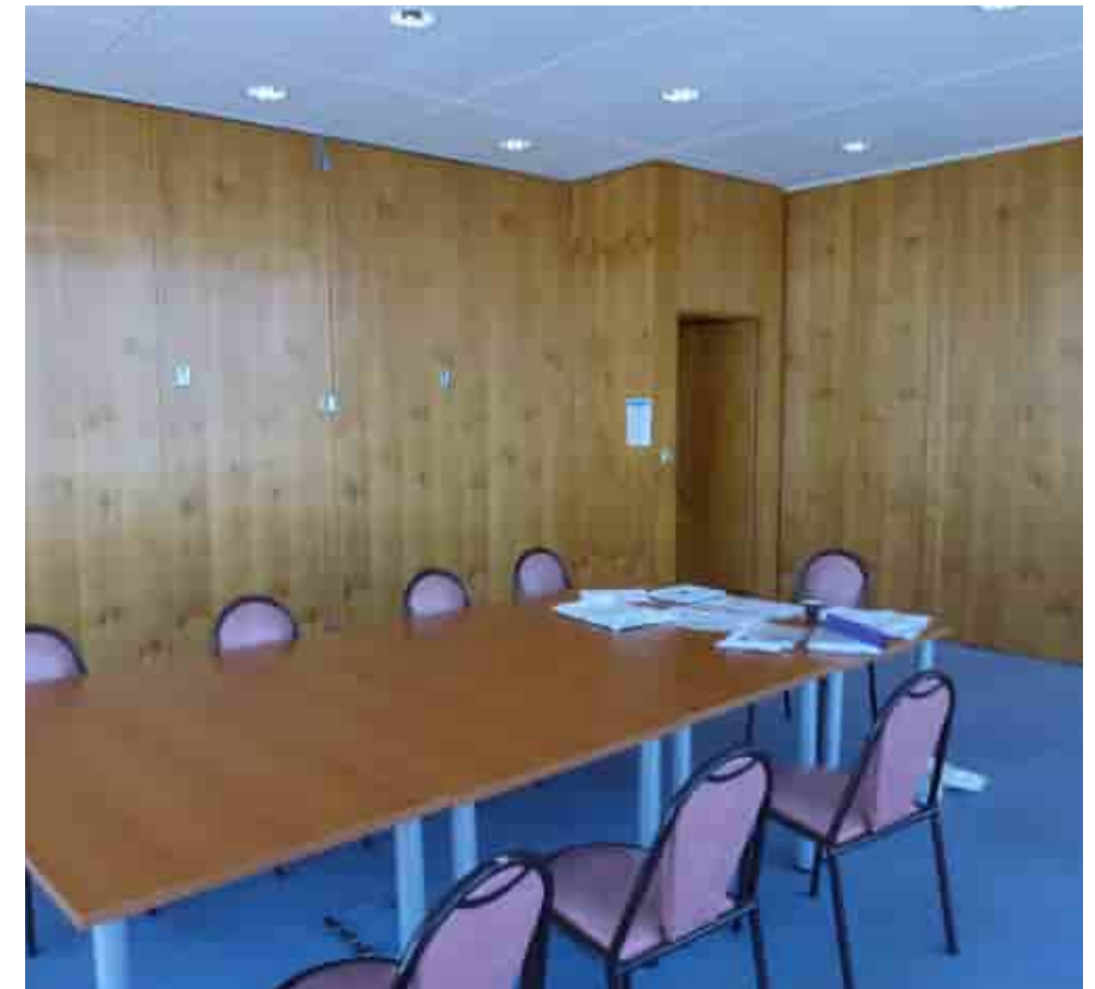
L24 cellular meeting room existing condition
