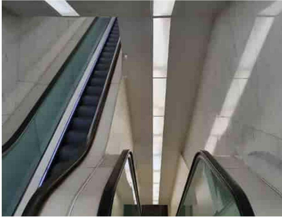
Current view of escalators- partial marble wall finishes
