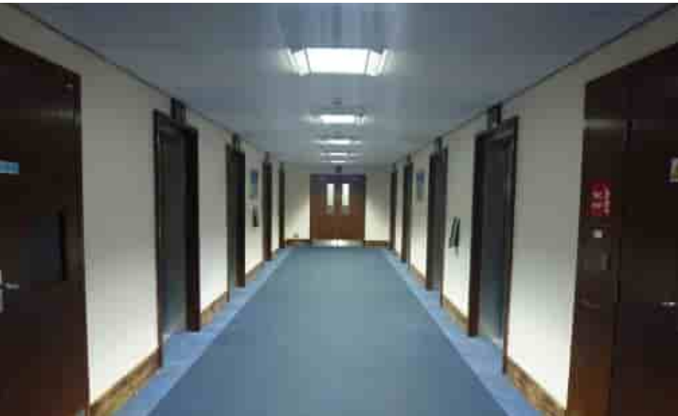
Existing lift lobby condition
