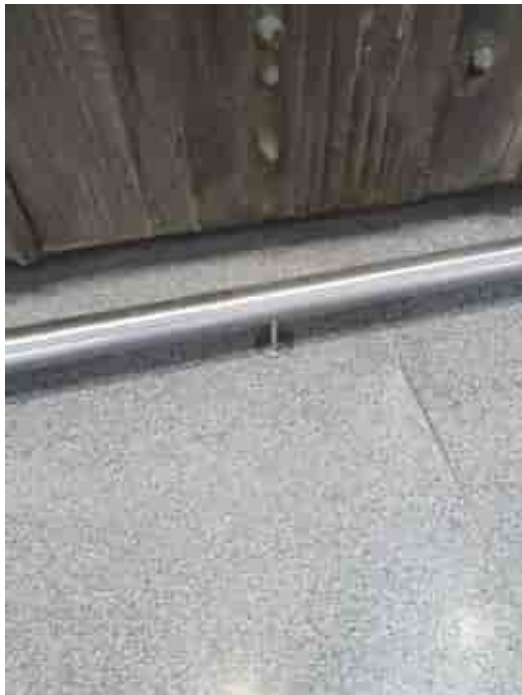
Rail fixed to floor
