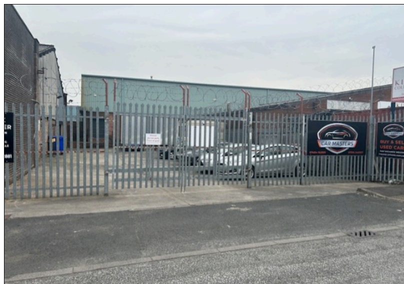
View of application site from Bradstone Road
