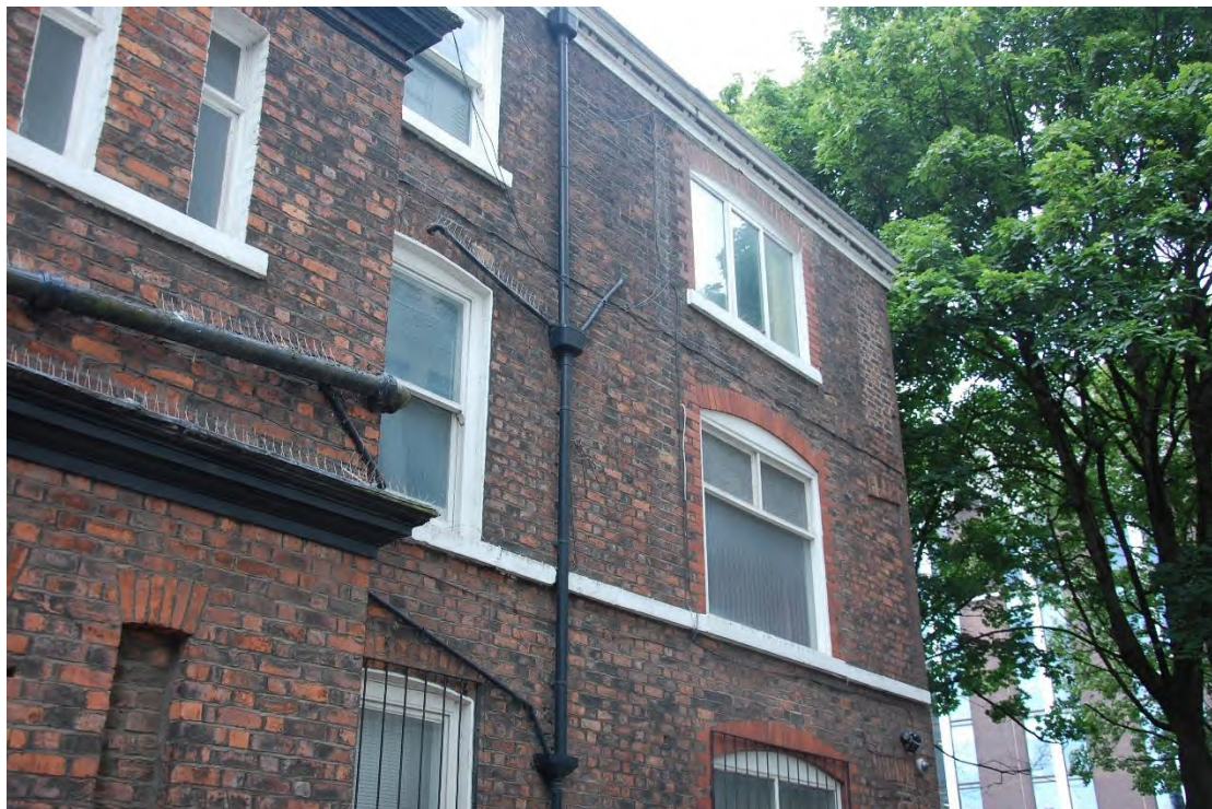
Photograph 2: Point of joining between 8/8A St John Street and old workers' terrace (bisected window noted by red arrow), looking north-west
