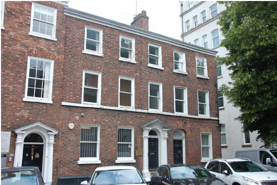
Photograph 3: 8/8A St John Street Façade, looking north
