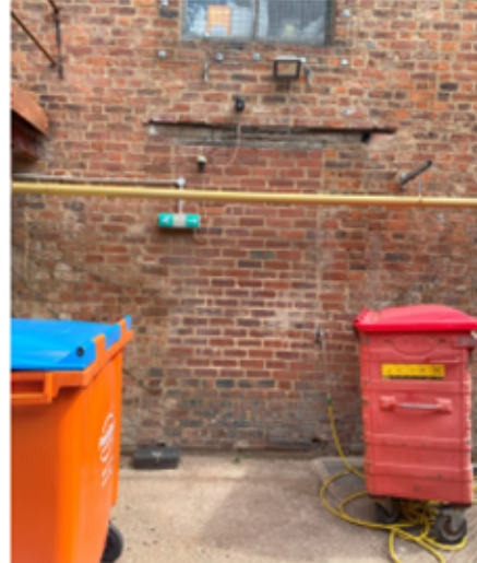
Existing bricked up fire escape door
