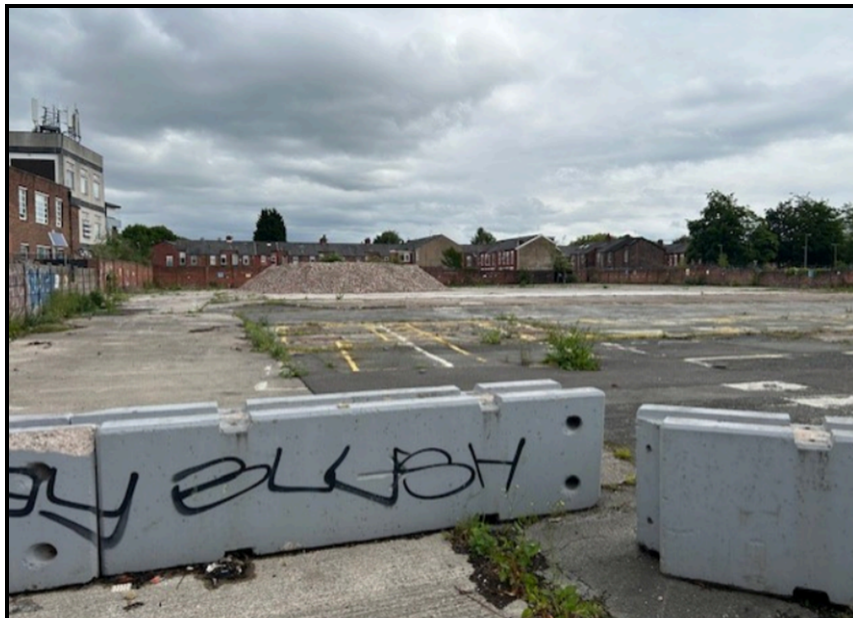
View of site from behind access gate on Wilmslow Road
