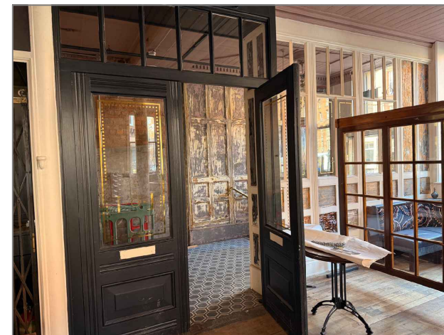
IMAGE REF 8: LOBBY DOORS & GLAZED / TIMBER SCREEN
