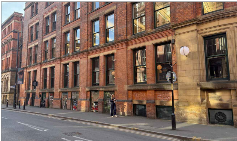
IMAGE REF 3: DALE STREET FASCADE
