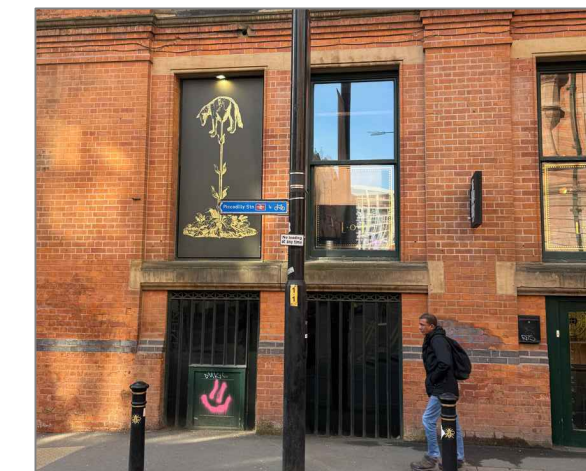
IMAGE REF 24: DALE STREET FASCADE - KITCHEN WINDOWS
