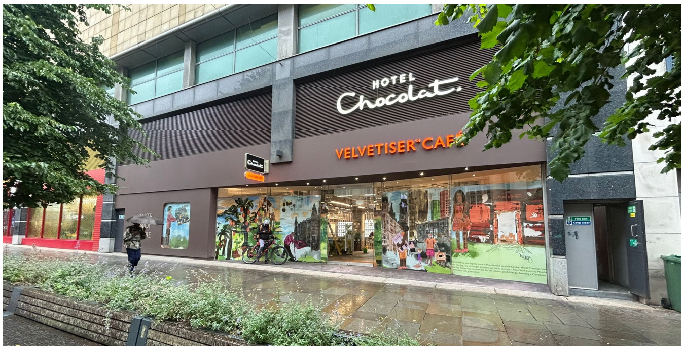
Figure 3 – Photograph of as built shopfront
