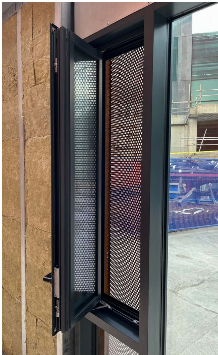
PPC Aluminium Inward Opening Window Colour: RAL 7016 Anthracite Grey
