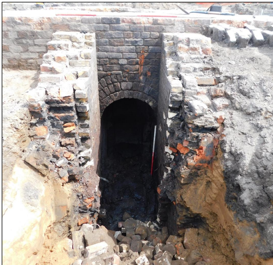
Plate 23: Flue 026 in the south-west of chimney 005, bounded by structure 008, showing the depth of the flue
