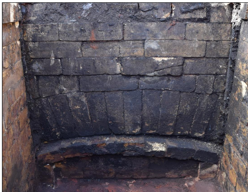
Plate 7: Wall [111], showing arch, looking south
