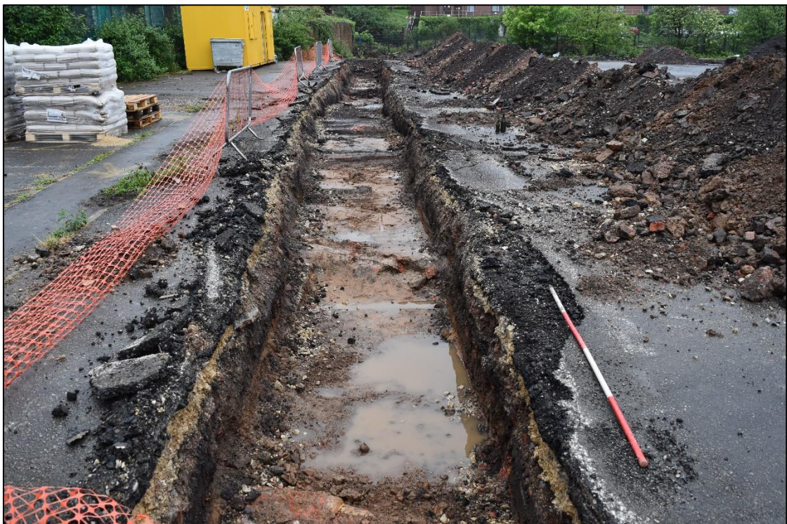
Plate 14: Trench 6, looking west/northwest
