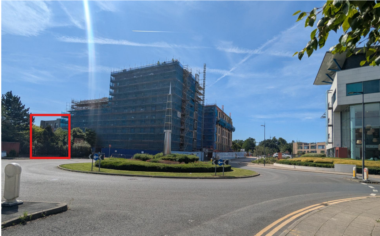
Photo of application site under construction adjacent existing part 4 storey residential building is identified in red to the left and the office building at One Didsbury Point is to the right
