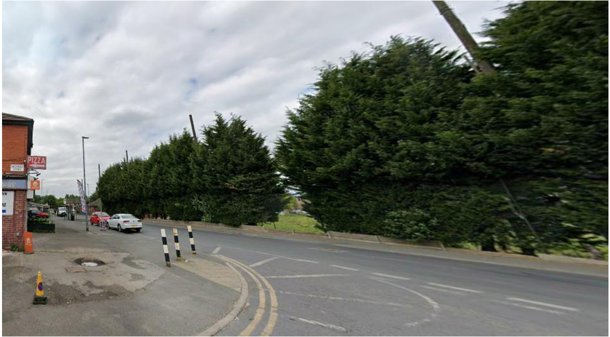
View of site from the junction of Mauldeth Road and Avonlea Drive
