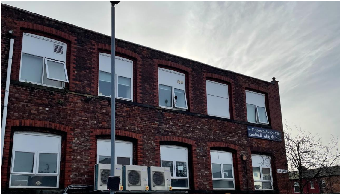
Figure 2 Photograph of unattended logger location 'L'
