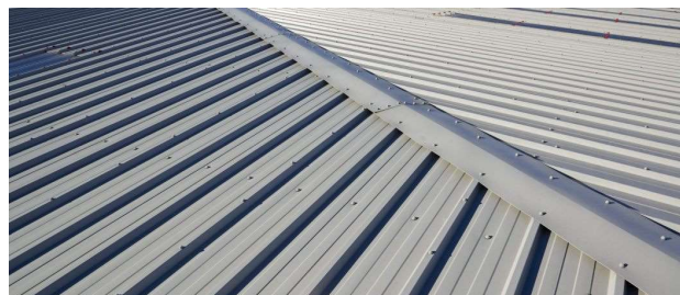
Roof to include canopies— Trapezoidal profile in Goosewing Grey
