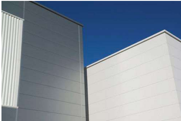
MicroRib composite panels horizontally laid. White RAL 9003
