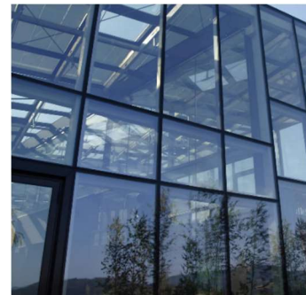
Aluminium Framed, PPC Finish Anthracite RAL 7016 – Double Glazed Infill
