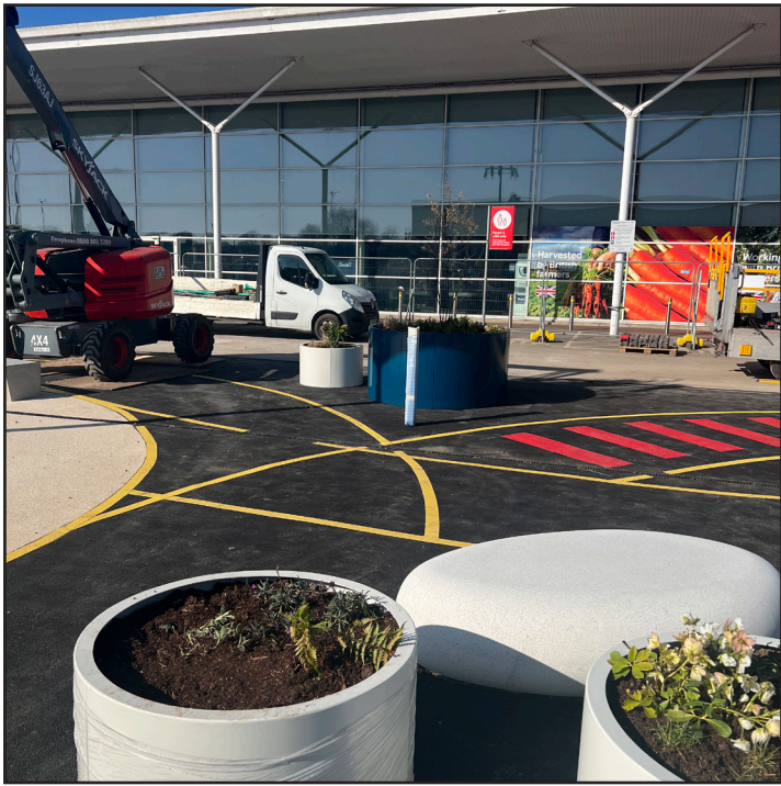
Figure 6 - Gorton Public Square - Continuation of Public Realm by Tesco Façade.
