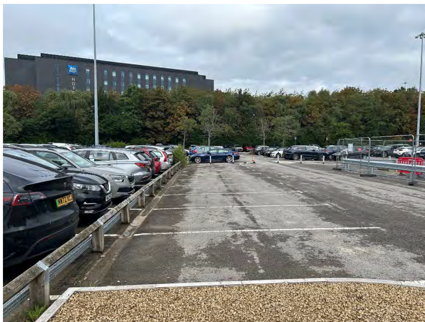
View west along southern boundary
