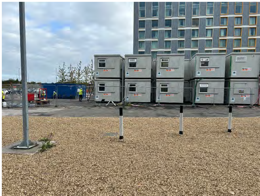
View north from southern boundary
