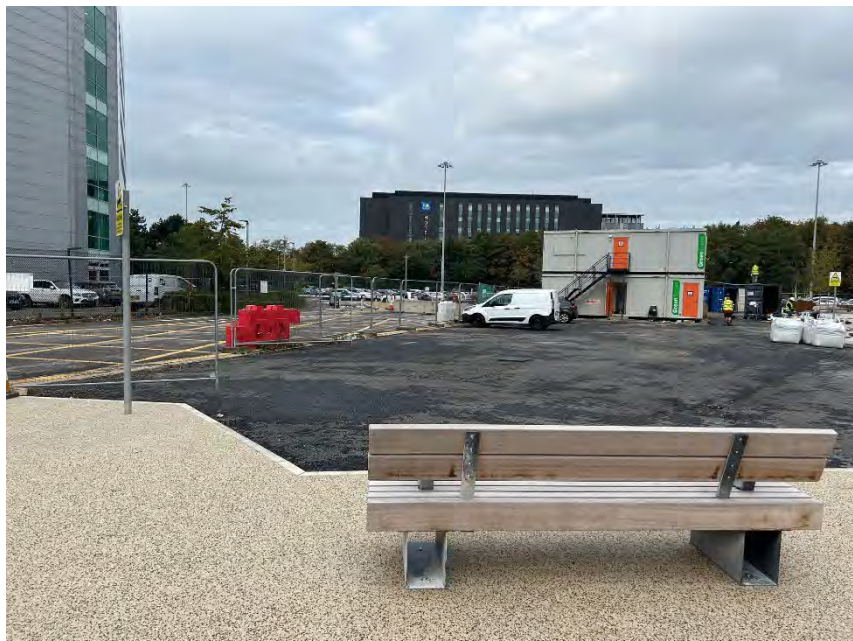
View west from eastern site boundary
