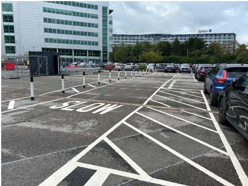
View south from western boundary
