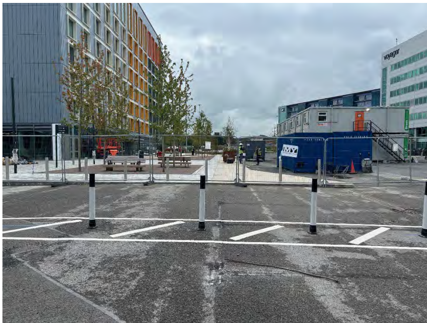
View west from eastern site boundary
