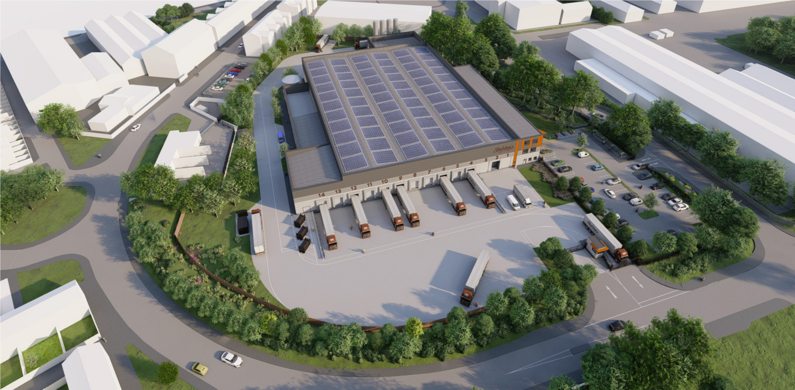
Overhead view from the south
