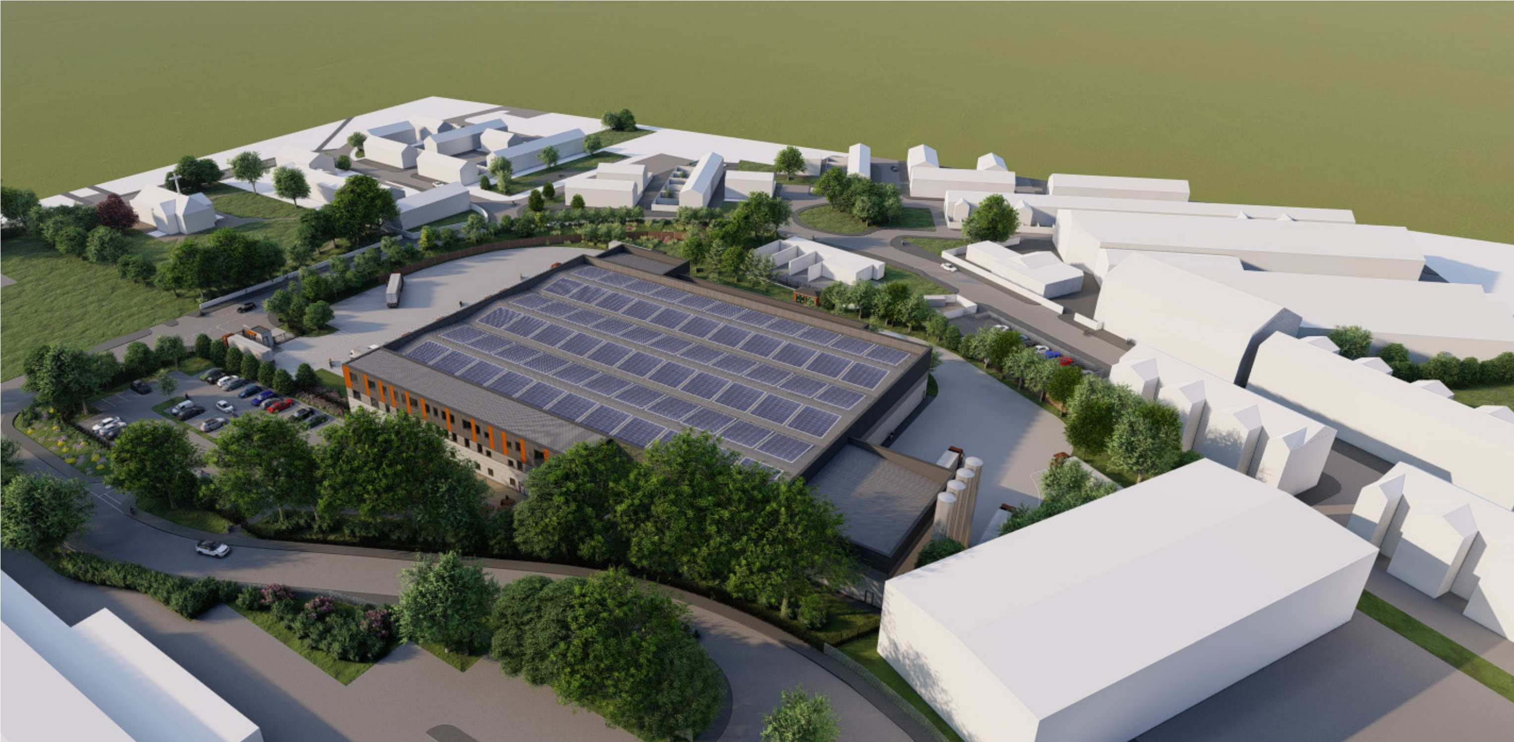
Overhead view from the northeast
