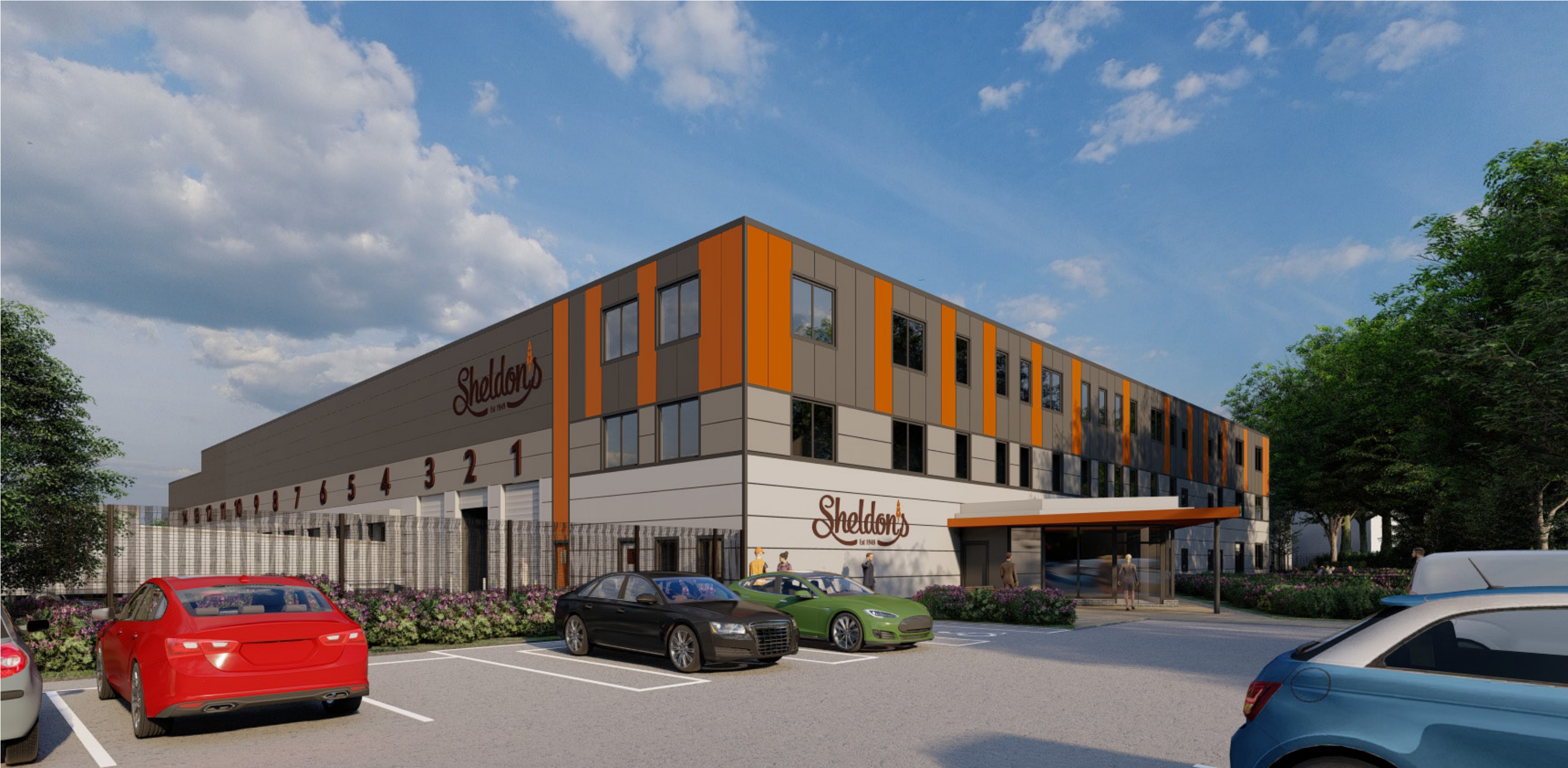
View towards main entrance
