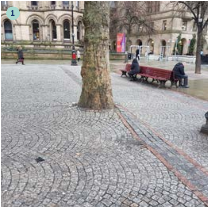
Granite setts to centre of Albert Square
