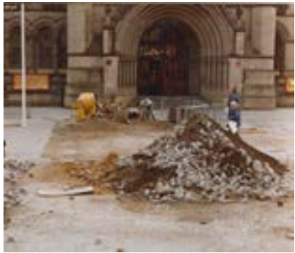
Granite setts being laid during the 1987 redesign
