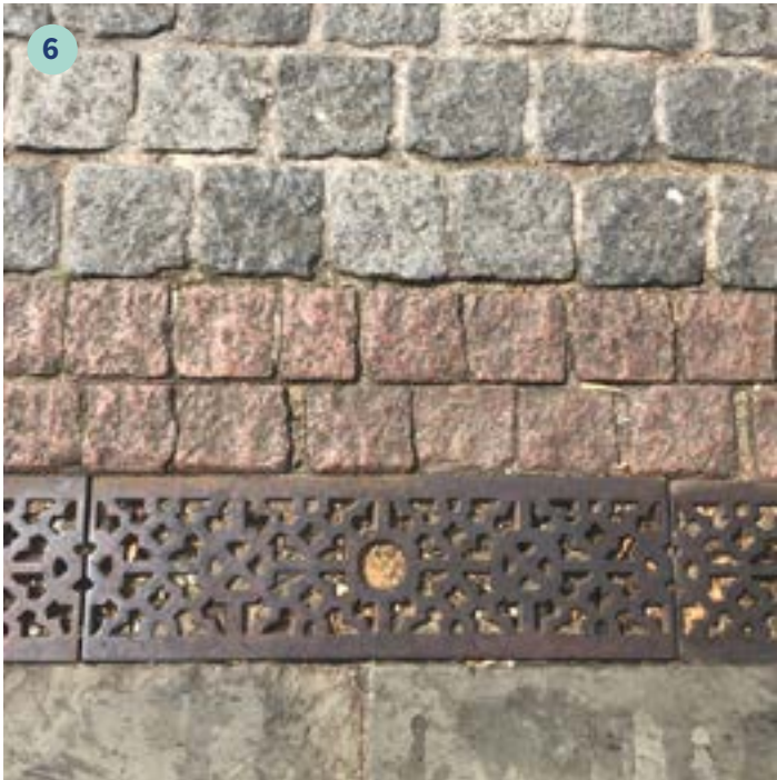
Metal grate edging detail separating Yorkstone flags and Granite setts to the edge of Albert Square
