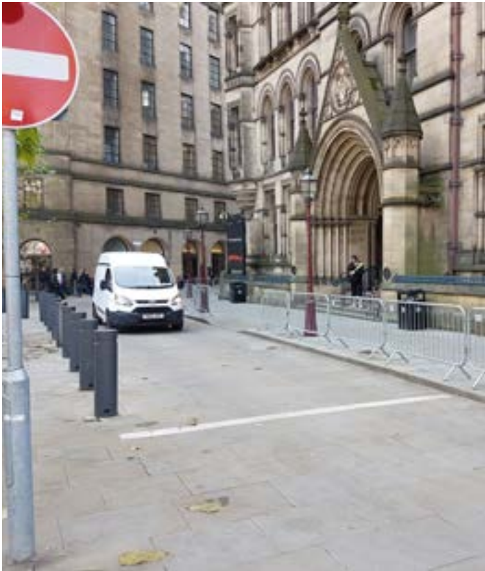
Image showing lack of barrier on Lloyd street
