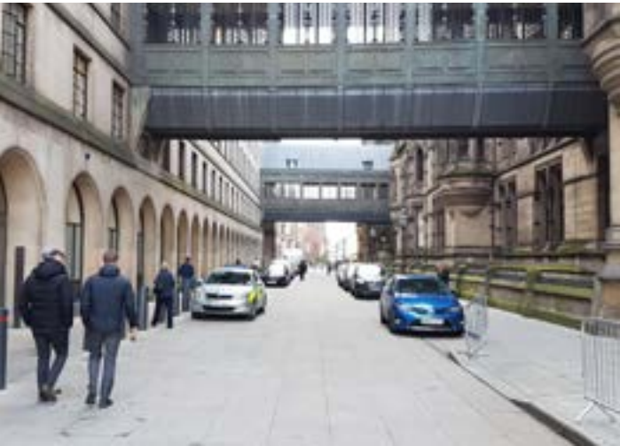
Existing Lloyd Street with little contrast between kerb and adjacent surfaces
