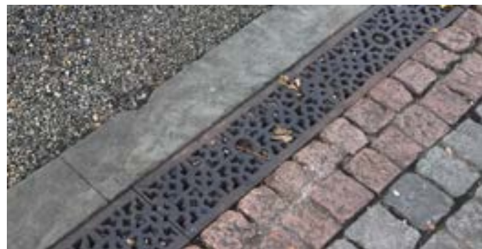
Existing Decorative Grating to Drainage Channel
