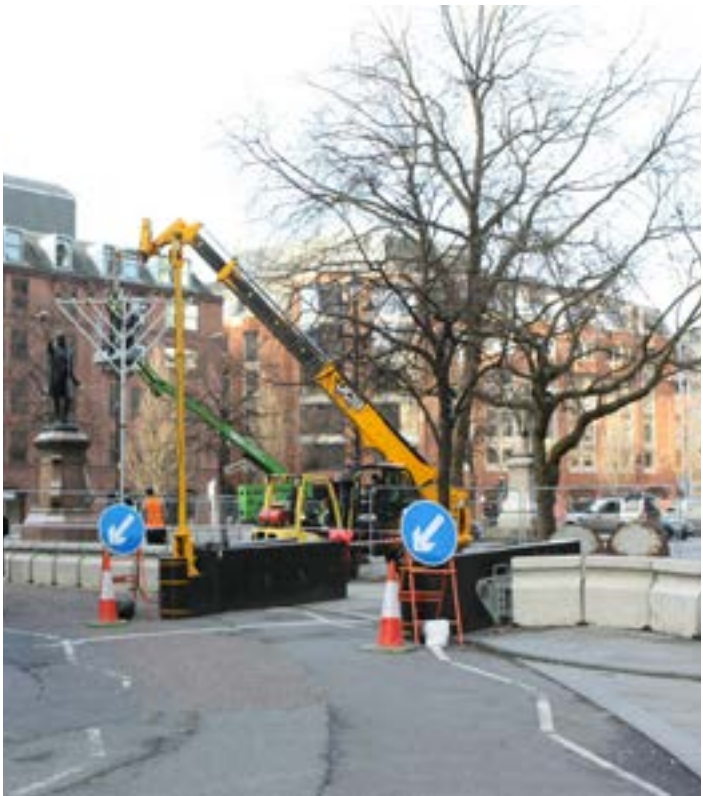
Image showing current HVM barrier to Albert Square
