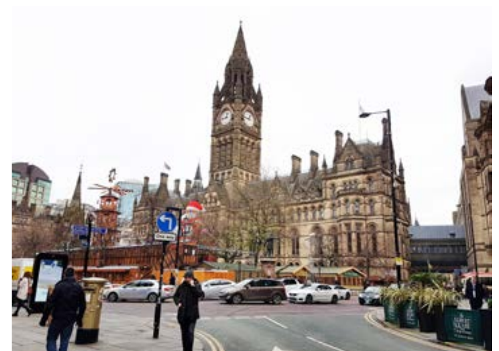
Current road creates a barrier and impacts upon the setting of the Town Hall
