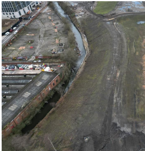
Figure 5 Photo showing existing condition of the river wall and embankment at the extents of the riverside footpath - facing downstream along the River Irk from the top of the river embankment
