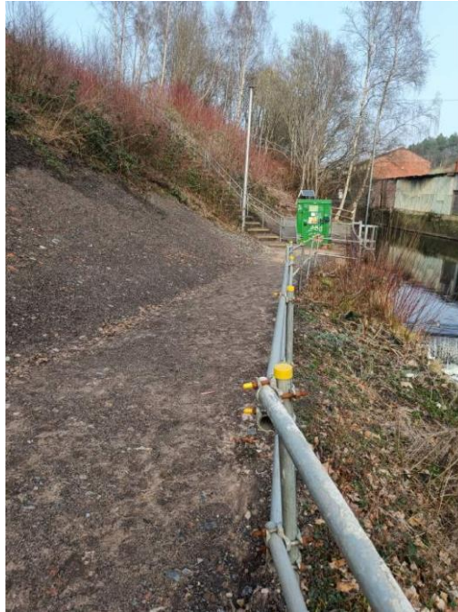
Figure 6 Photo showing existing condition of the 'EA Footpath' with temporary balustrade installed during construction works
