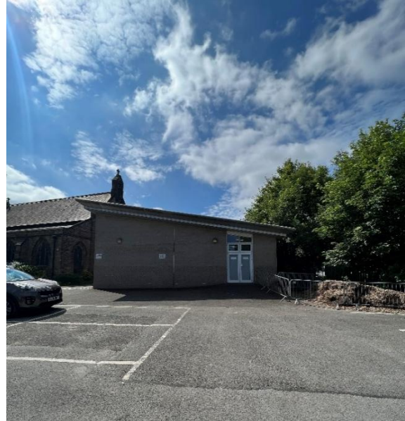
Figure 16 - View of Existing Extension
