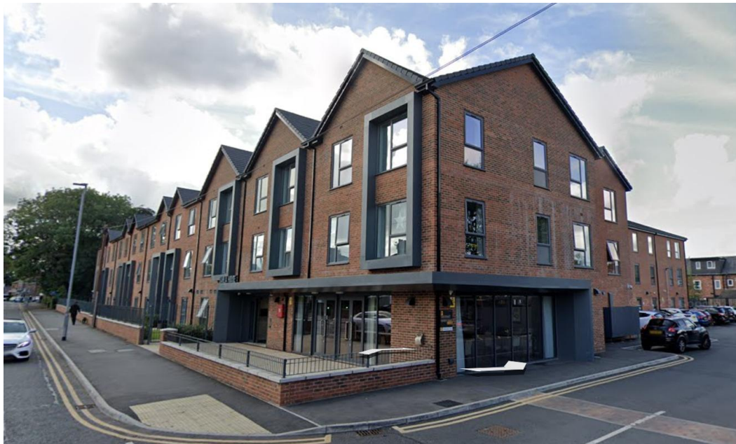
Figure 12 - New Apartment Building
