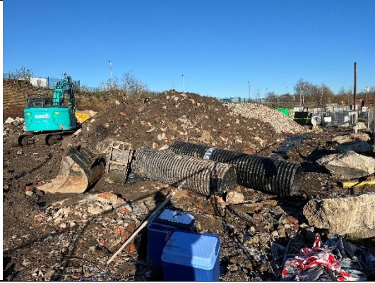
Photograph 5: View of stockpile of contaminated material excavated from Area 2.
