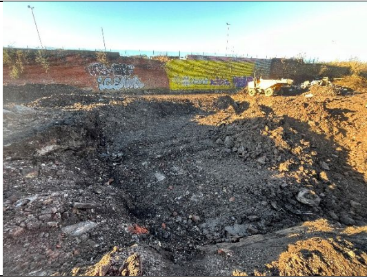
Photograph 5: View of extent of excavation area of Area 2 so far, rear of the photo has already been backfilled for safety.
