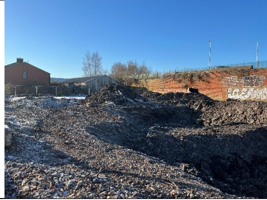
Photograph 6: View of stockpile of contaminated material excavated from Areas 1 and 2.
