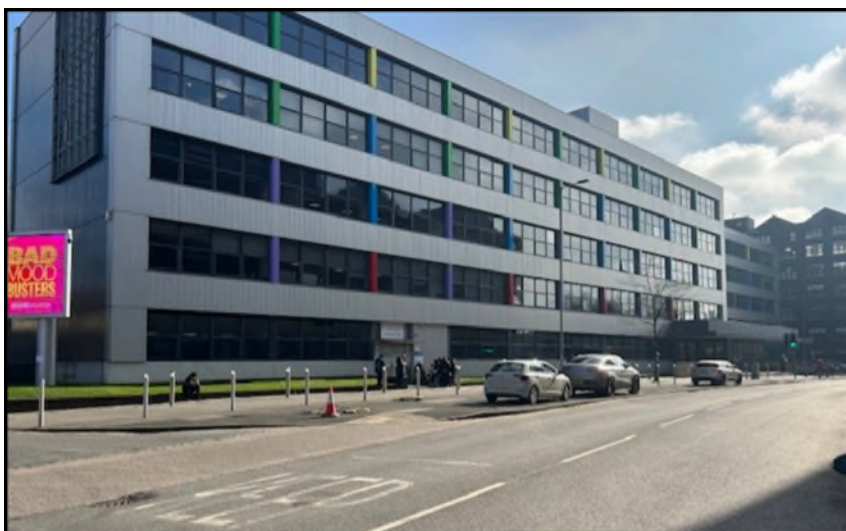
View of application site
