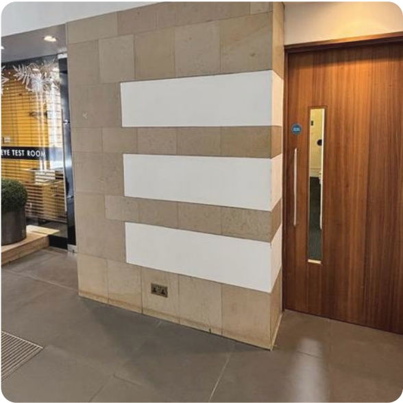
Existing Lobby Panels
