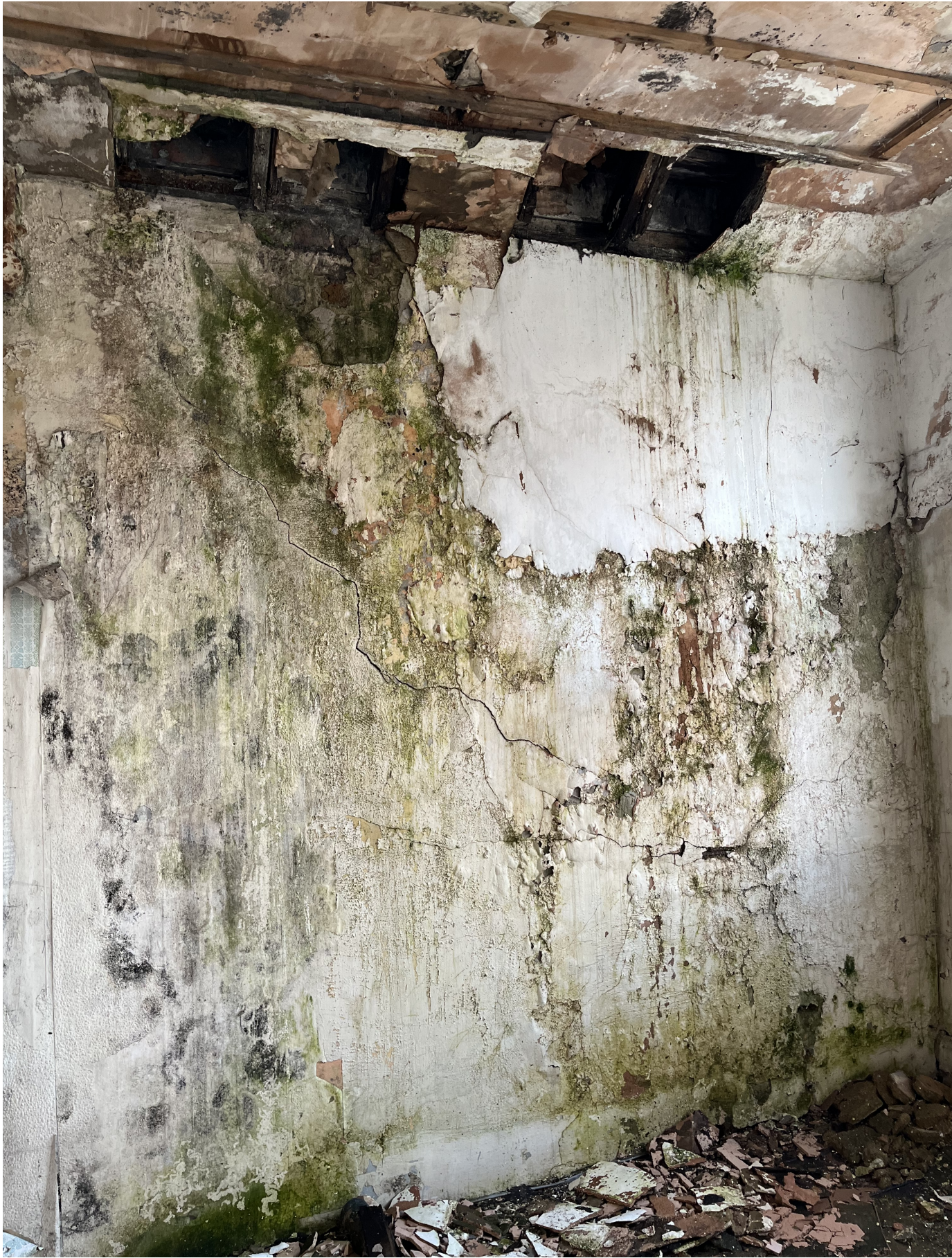
IMG_0458 (Second Floor - Internal dividing wall from No.70 side)
