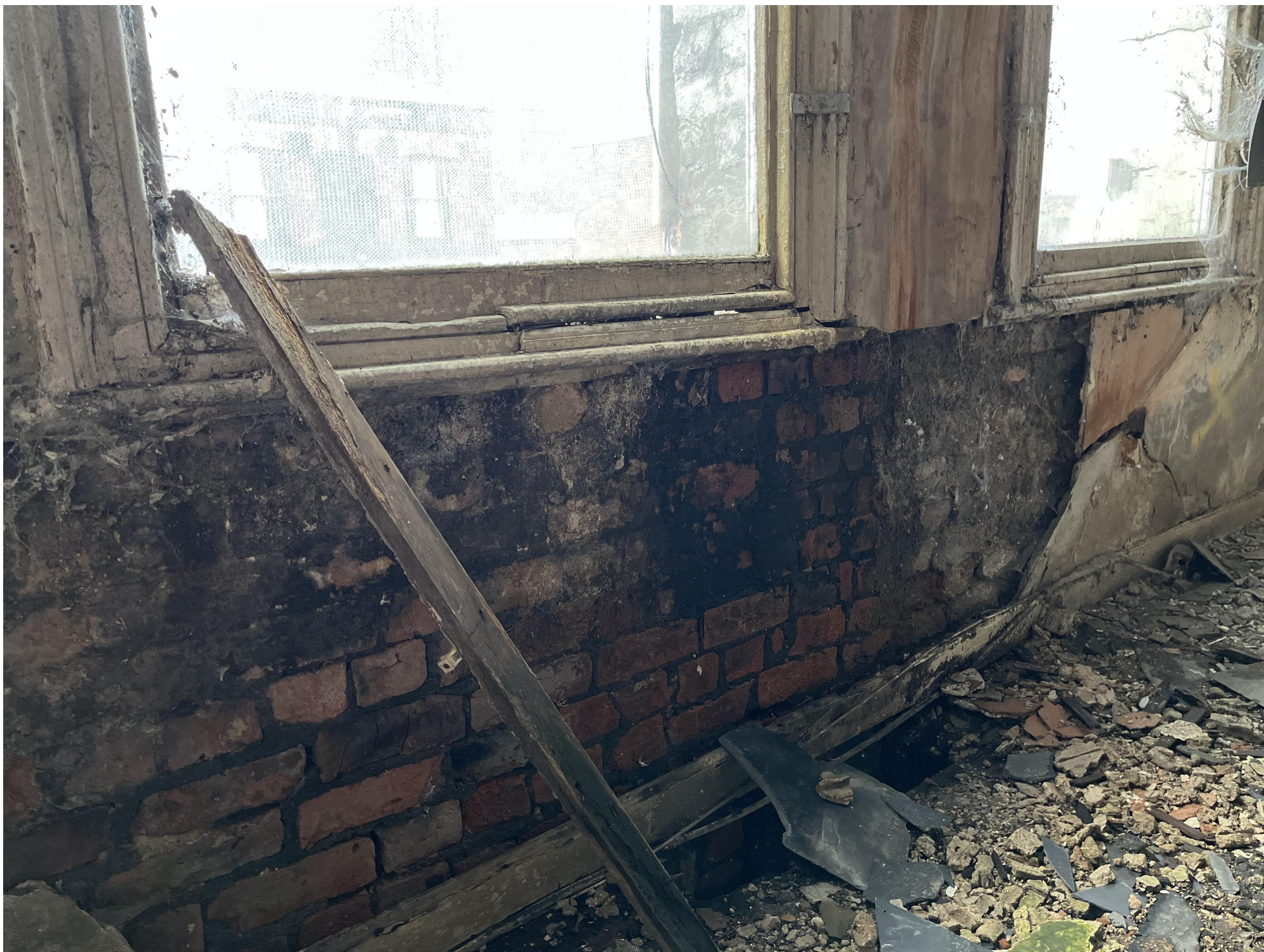
IMG_0446 (Second Floor - No.68 facade)
