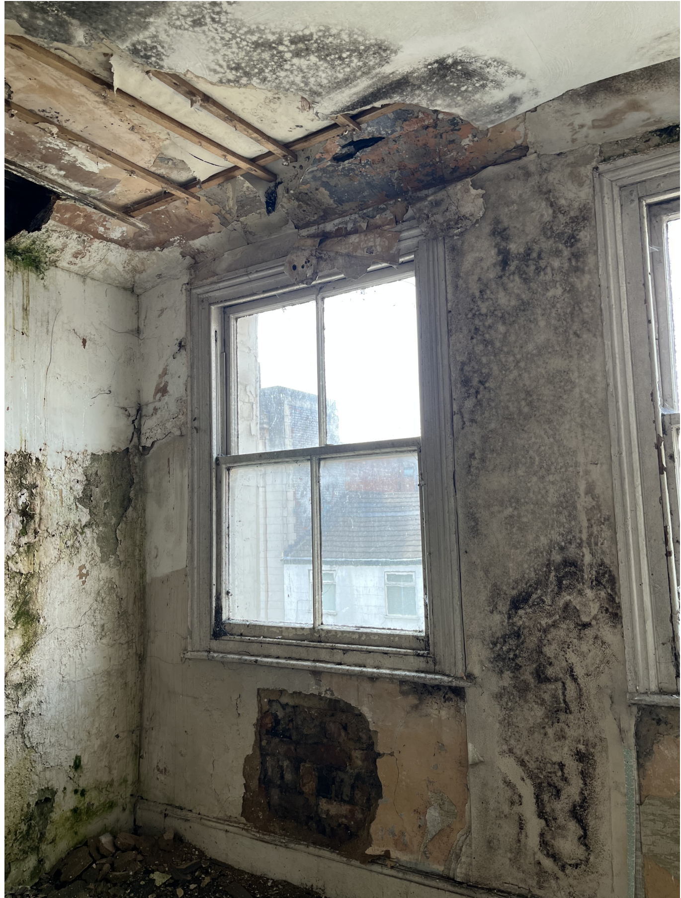
IMG_0459 (Second Floor - No.70 facade)
