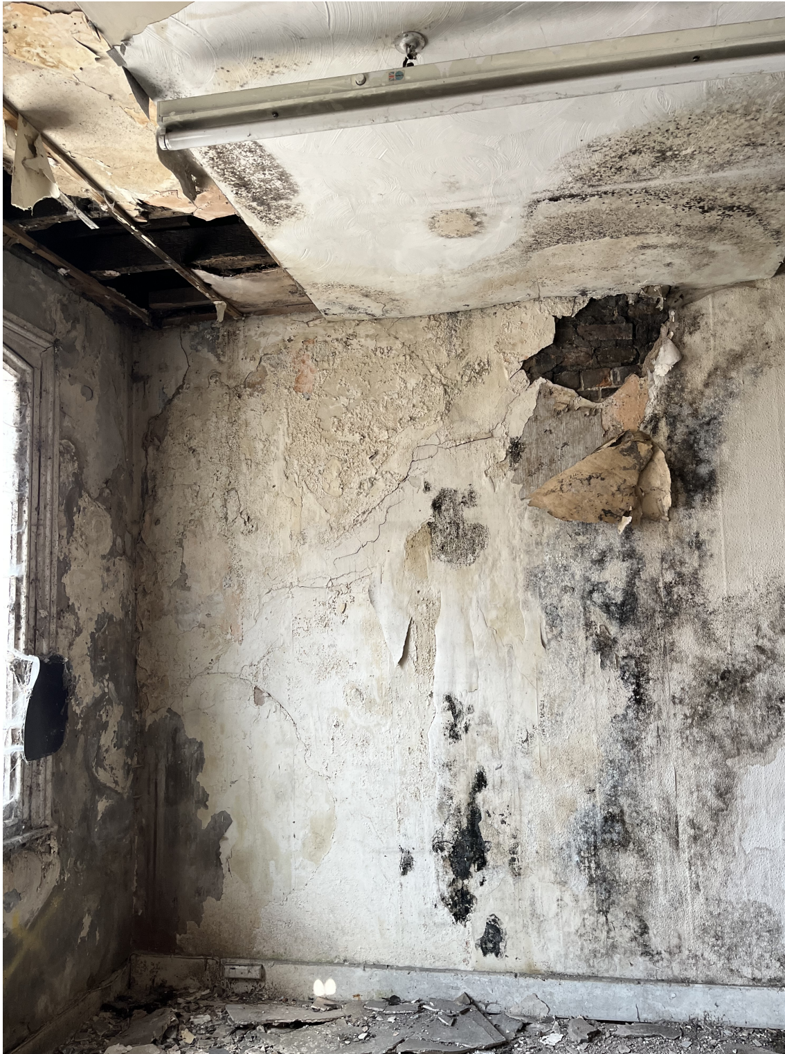
IMG_0450 (Second Floor - Internal dividing wall from No.68 side)
