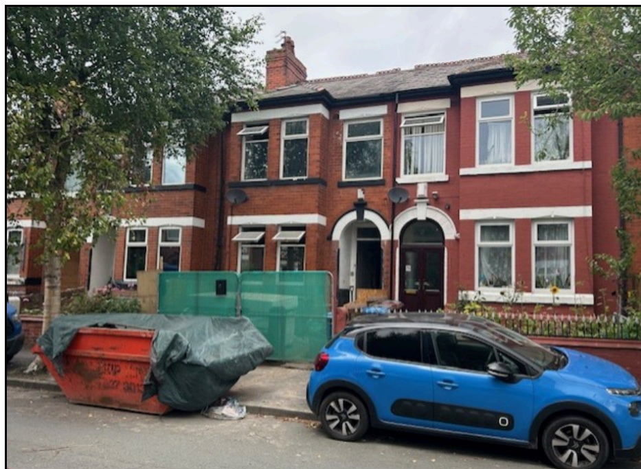
View of application property from opposite side of Langdale Road
