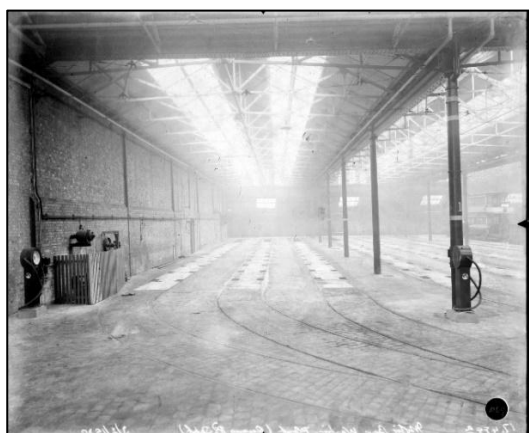
Figure 27: 1930 photograph of the Bus washing plant within Queens Road Bus Depot. This was built to support the influx of motorbuses that Manchester Corporation had acquired. Source: City Engineers Department, Greater Manchester Lives Archive
