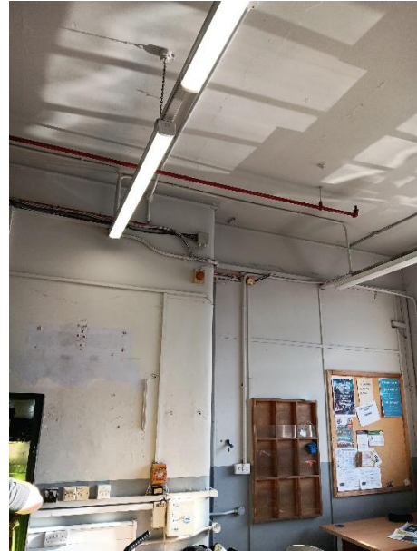
Figure 21: Partition as seen from Drivers' Mess (GF.01), with chimneybreast to the left of the frame.
