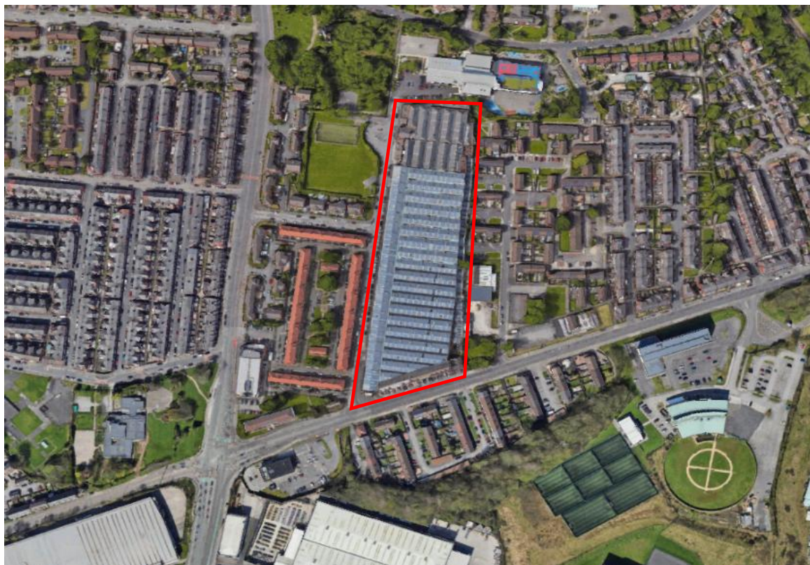
Figure 1: Aerial view of the Queen's Road Bus Depot, illustrating the scale of the full site. Source: Google Earth.
