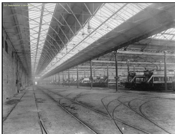
Figure 26: 1902 Photograph of the interiors of the electric tram shed. Source: Greater Manchester Lives Archive
