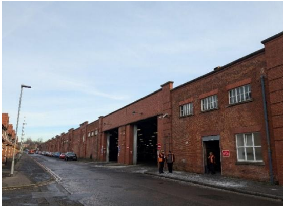
Figure 6: View of the Boyle Street elevation, showing the red brick, utilitarian characteristics with modern openings for buses.
