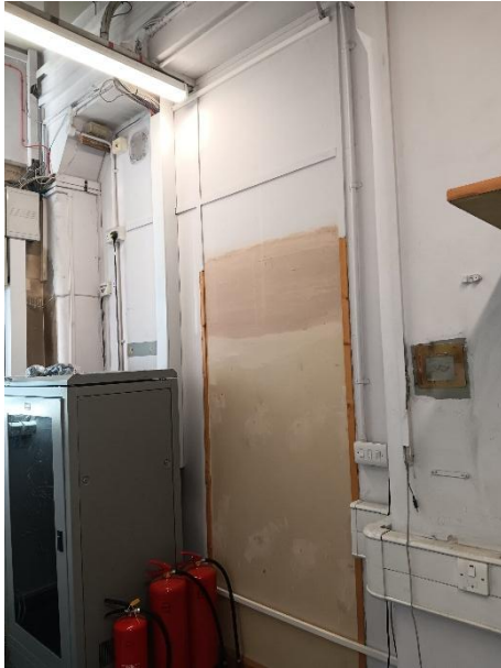
Figure 20: Infilled opening between Reception (GF.02) and Drivers' Mess (GF.01), to south of existing chimneybreast.
