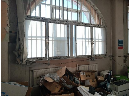
Figure 14: Security fixtures attached to interior of windows, Money Drop Office (GF.07).
