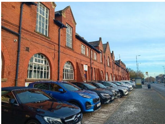
Figure 8: Queens Road frontage, which includes public reception entrance.
