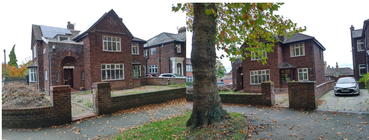
Fig.1 – Views of the site from Errwood Road
