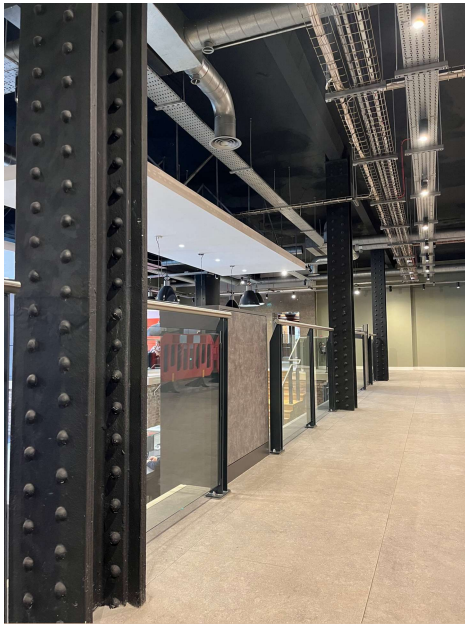
Existing steel & glass balustrade
