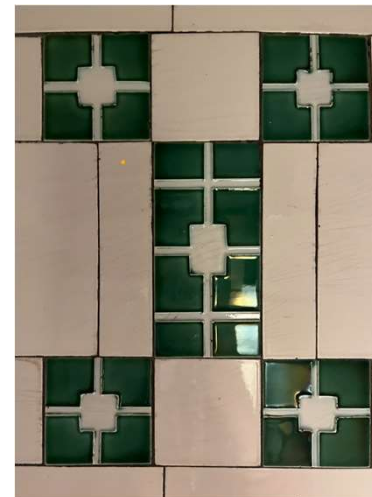
Existing decorative wall tiles in basement
