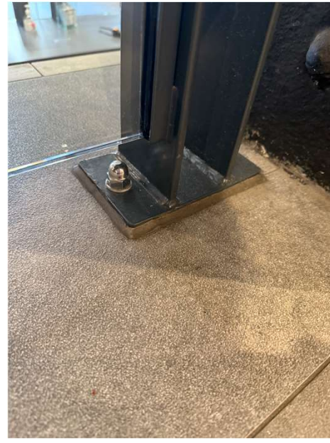
Existing balustrade fixing detail
