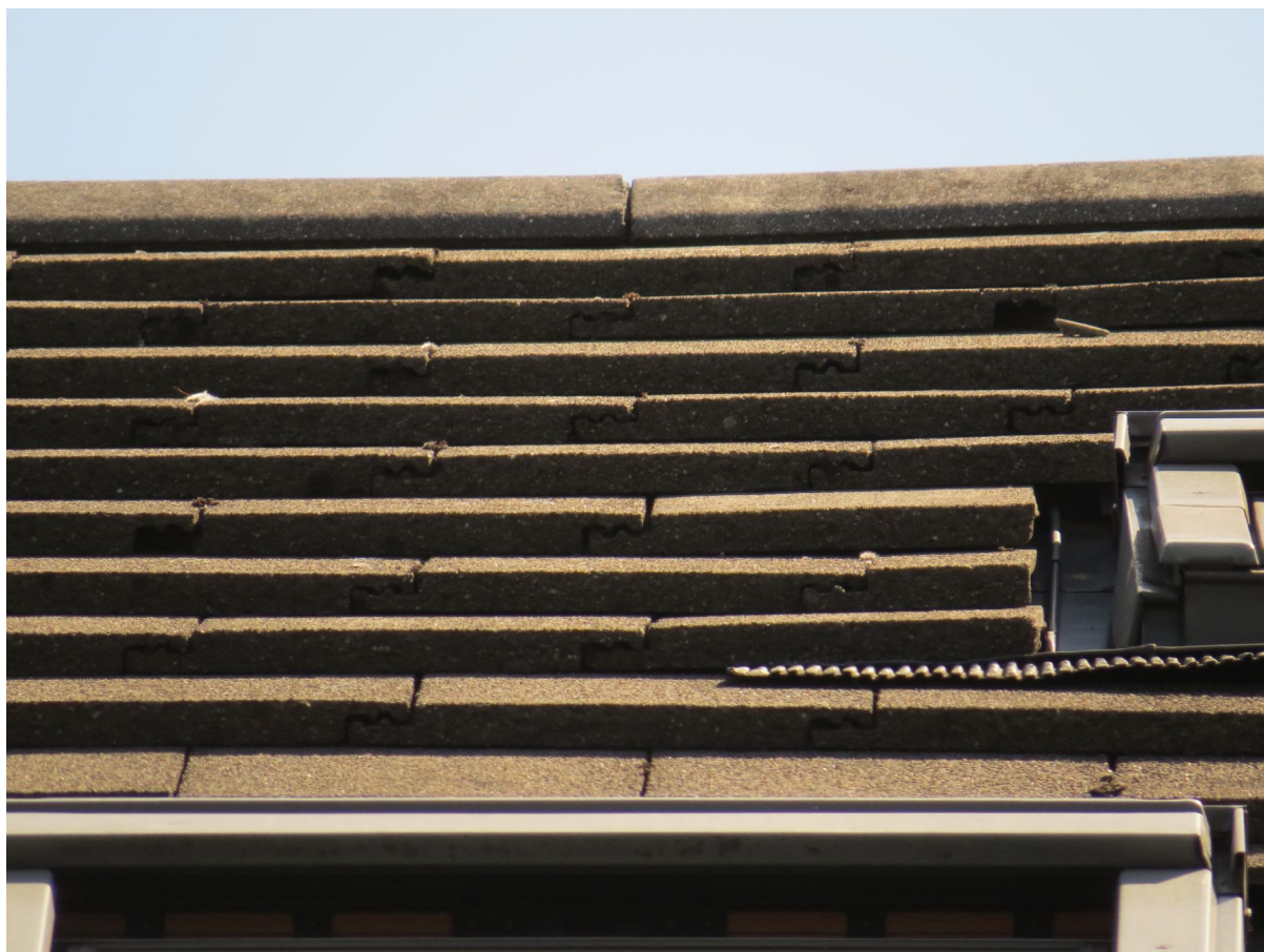
6 – The roof and ridge tiles of Nº17 are tightly fitted with no suitable gaps.
