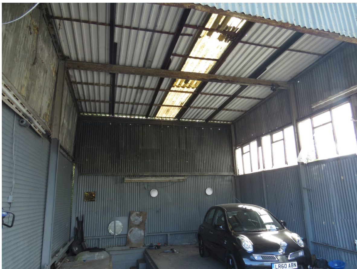
3.1a – The open sided steel shed to the rear of N°17.
