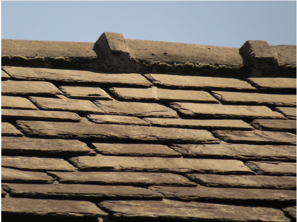
7 – The roof and ridge tiles of N°19 are tightly fitted with few gaps..
