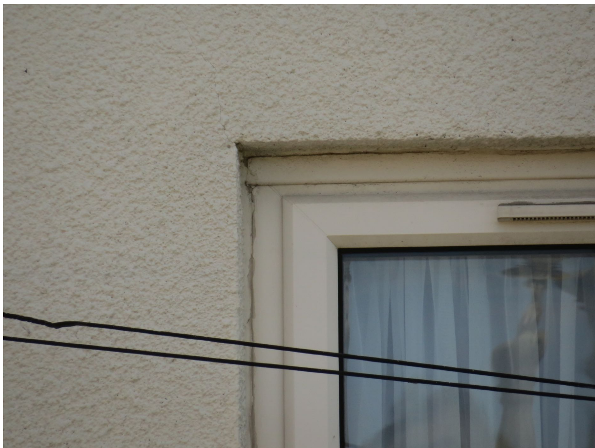
10 – UPVC window frames are tightly fitted.
