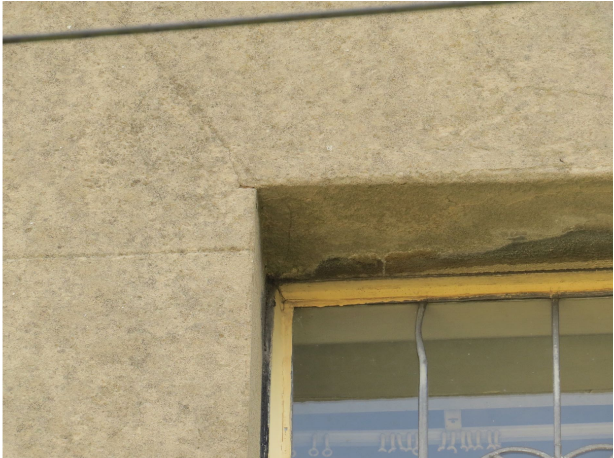
11 – Timber window frames are tightly fitted with no gaps between frames and brickwork.
