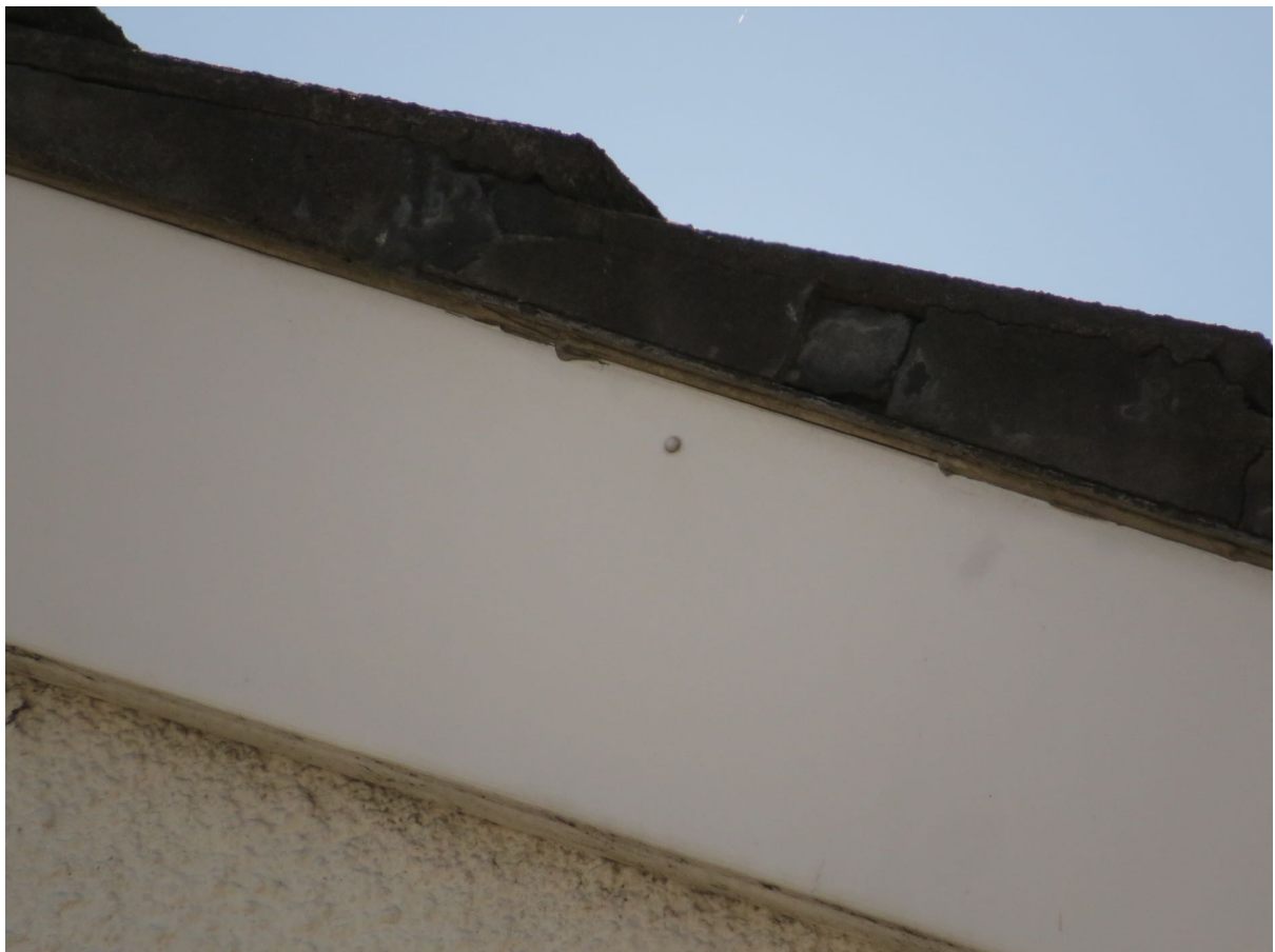
8 – End tiles at the verges are sealed with cement fascias are fitted tightly.
