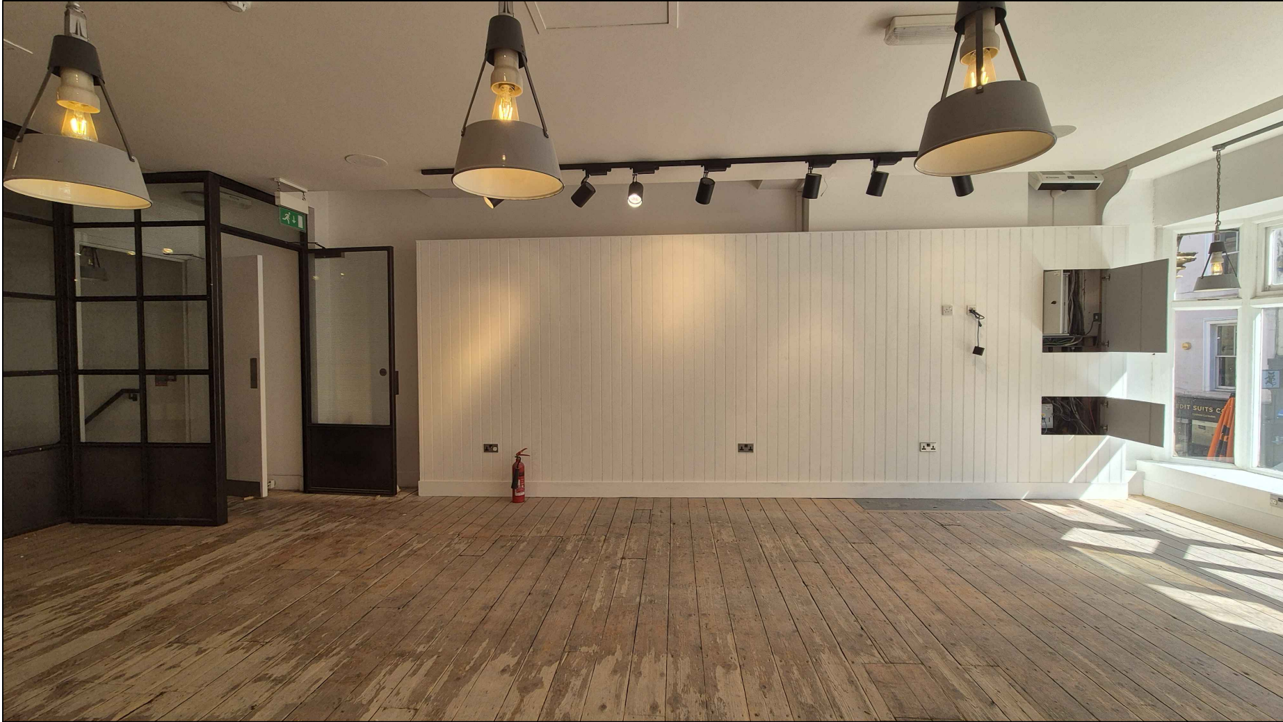
1st Floor - EXISTING - photo
