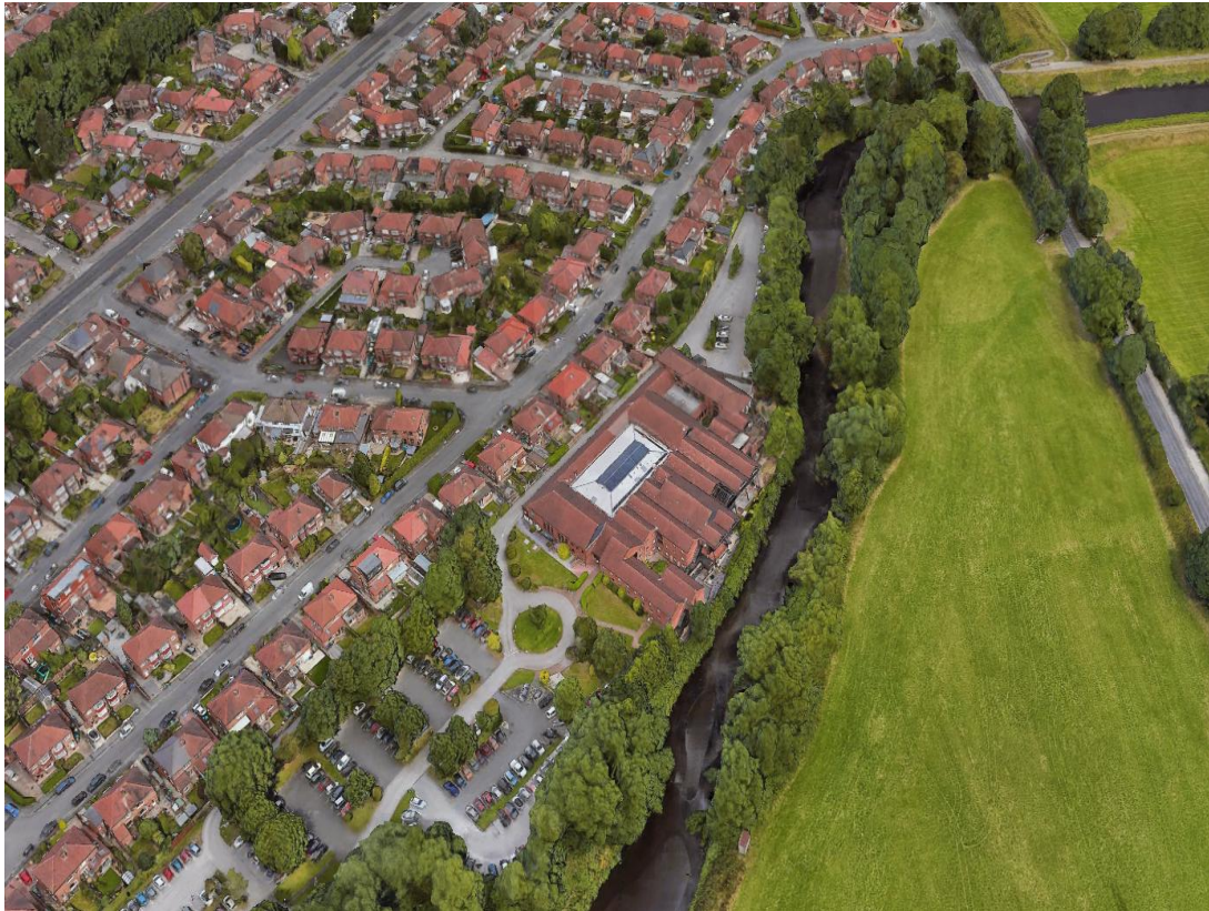
Image 2 – Overhead view of site facing northwards
