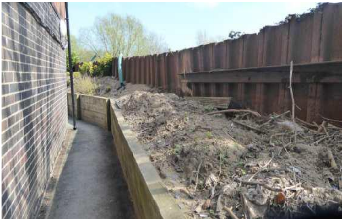
Image 5 - Photograph of existing flood wall adjacent to eastern boundary of the site facing northwards
