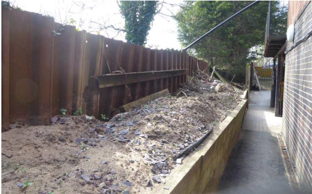
Image 4 – Photograph of existing flood wall adjacent to eastern boundary of the site facing southwards
